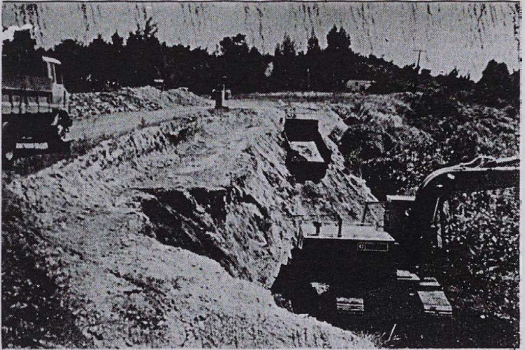
Contractors stabilising the outside edge of the car park
