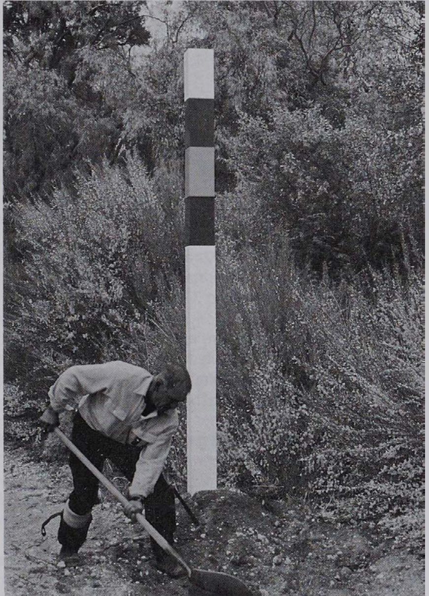
Compliance Officer Bryan Taylor erects another of the new 300-metre markers.
