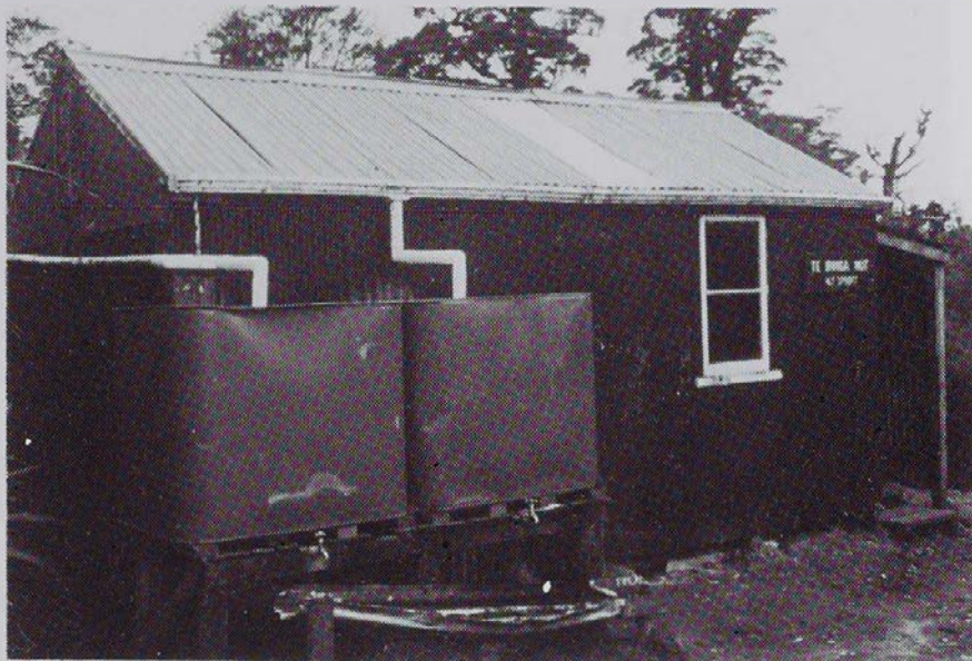
New water tanks at Te Iringa Hut.
