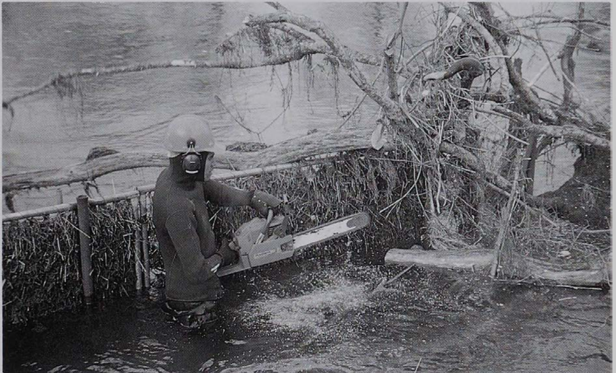
Conservation Officer Bonzo Ngamotu clears log debris off the lower Tongariro trap following floods in July.
