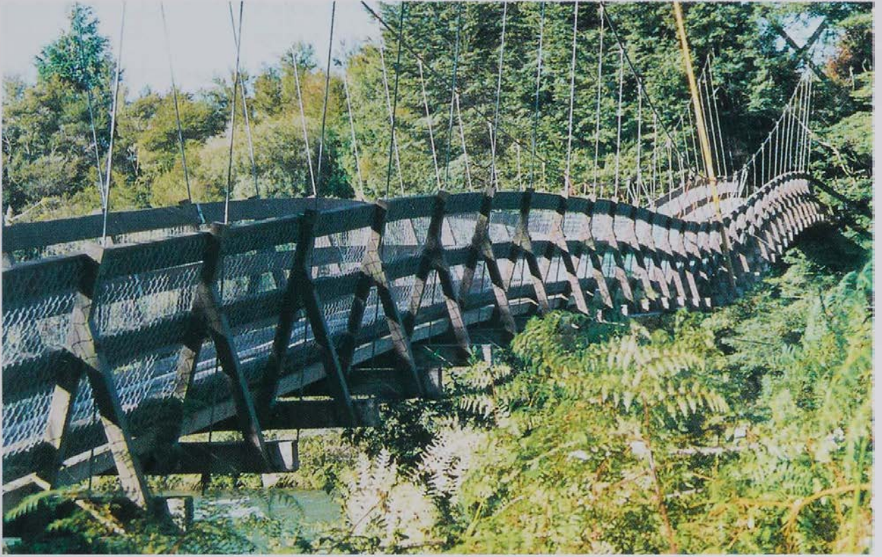
The bridge under a three tonne load.
