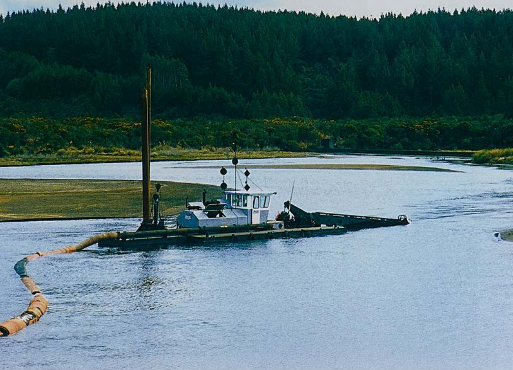
The cutter suction dredge operating in Lake TeWhaiiau
