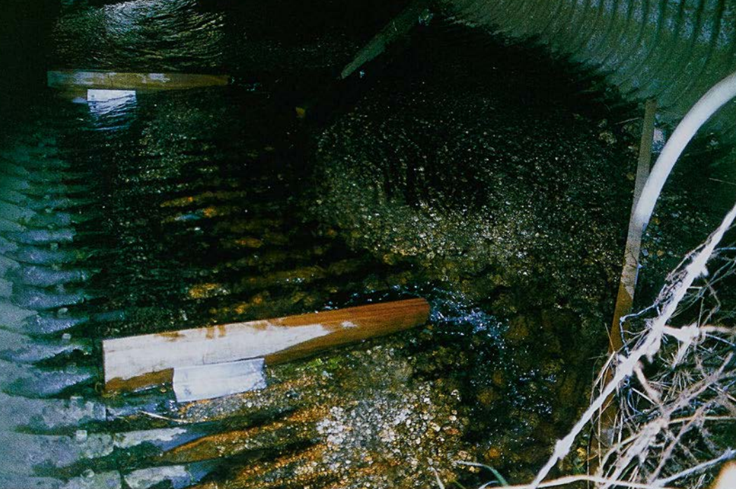
Above: Wooden baffles used to restrict and deepen the flow through a culvert. Photo Jon Palmer
