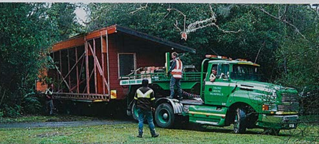
The lodge was cut in two in order to bring it through the trout centre. Although the route the removal trucks took was not the easiest, it meant minimal impact on areas of the centre that the public enjoy. Much thought was put into ensuring the least amount of damage was done to native vegetation and the aesthetics of the site. Photo: Petrina Francis
