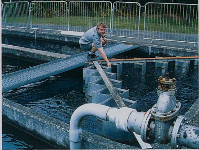
Callum Bouke checks the vanes that direct the water around the raceways Photo by: Kim Alexander-Turki
