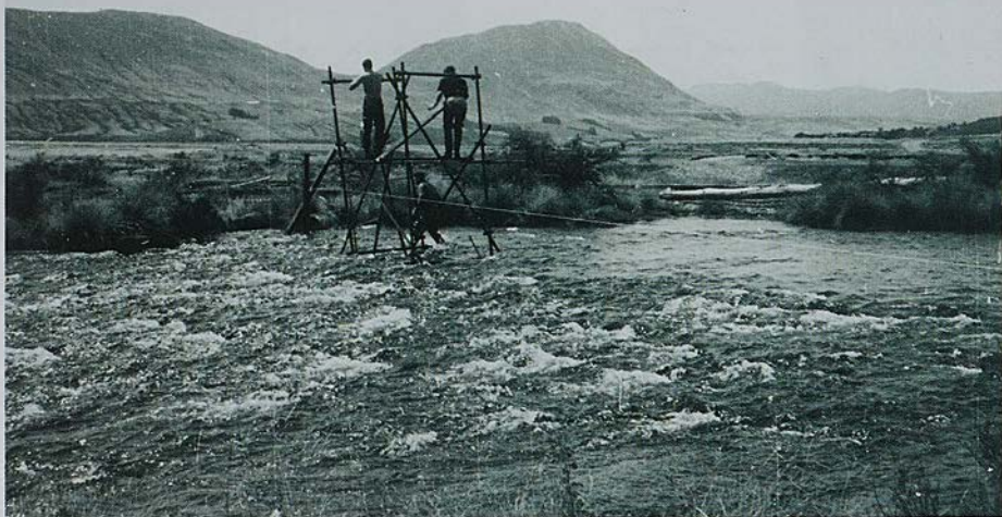
Driving railway irons to support the trap barrier in day's pre Health and Safety. Photo by: Errol Cuddy
