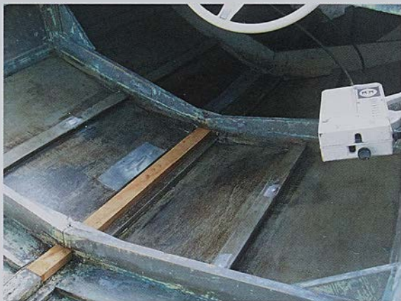
The interior was completely stripped Photo by Mark Venman
