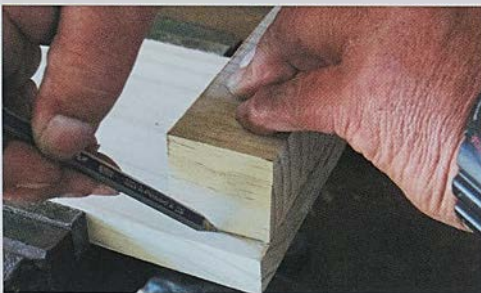
Mark the position of the block on the board Photo by John Webb
