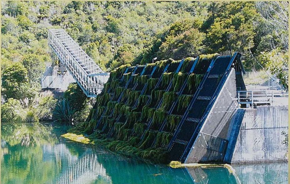
Removing hornwort before the Rotoaia intake. Photo courtesy of Genesis Energy
