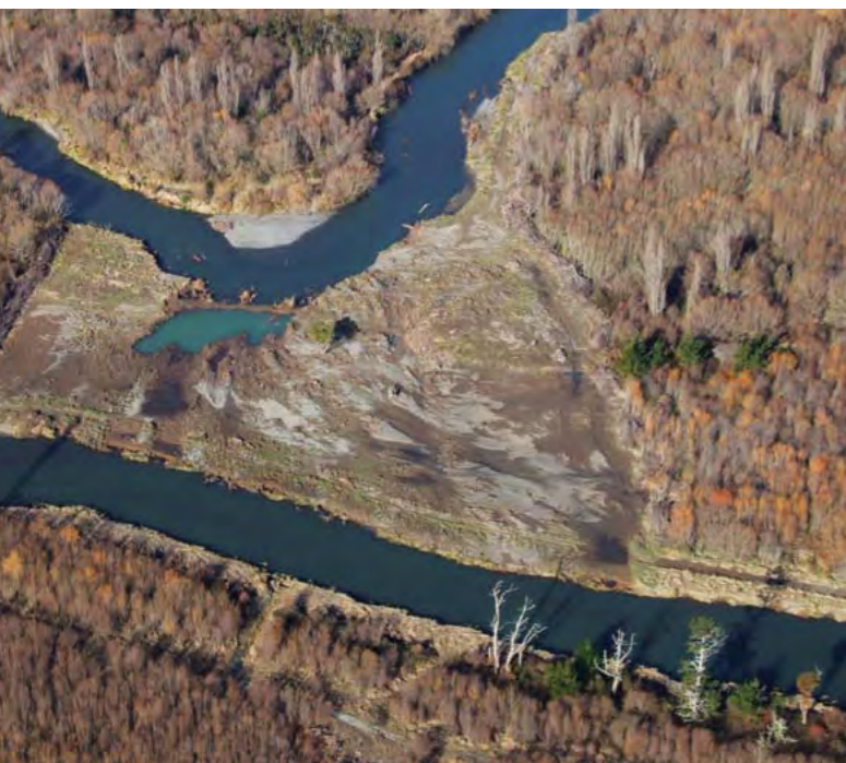
BELOW Aerial photo of willow clearance, delatours pool. Photo by Pete Shepherd
