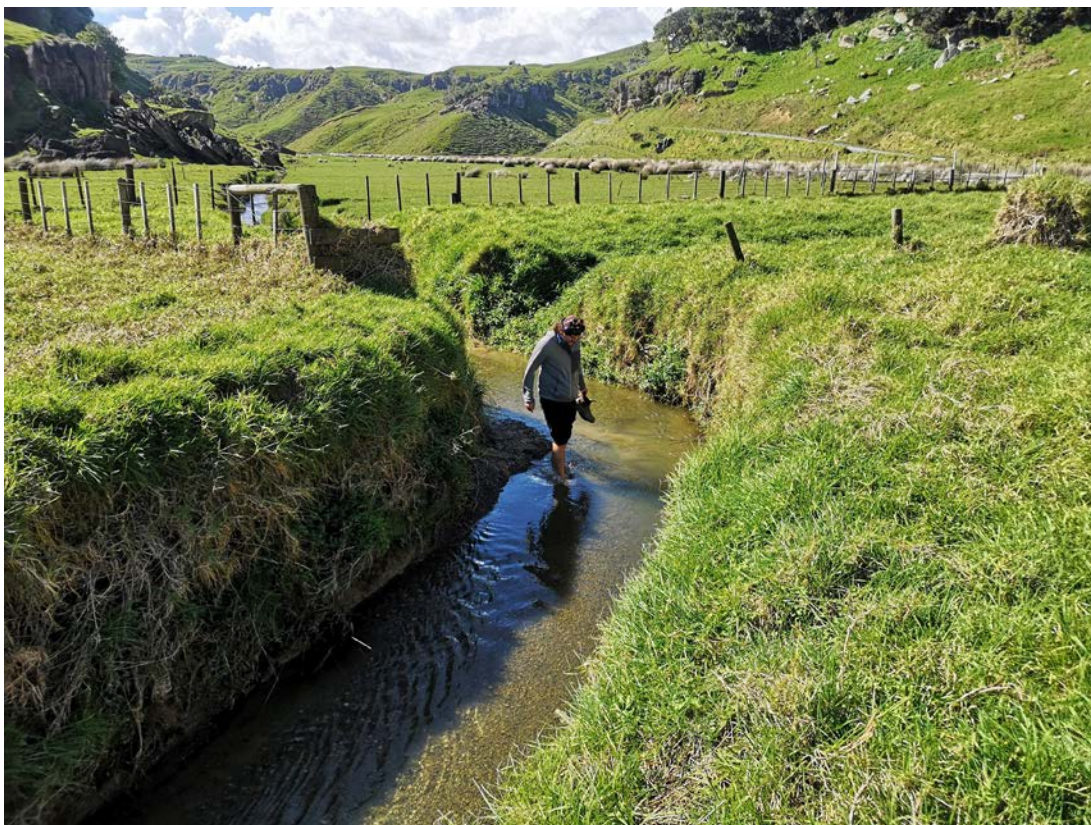
FIGURE 1-11 DRAINAGE CHANNELS ARE DESIGNED FOR OPTIMUM CONVEYANCE; STEEP BANKS ALLOW DEEP AND FAST FLOWS IN FLOOD EVENTS, EFFECTIVELY FLUSHING SEDIMENT AND DEBRIS ON RELATIVELY LOW SLOPES. CANALS ARE STRAIGHT, TAKING THE MOST EFFICIENT ROUTE AND TYPICALLY DIRECTING WATER TO THE MARGINS OF PRODUCTIVE LAND. THEY BEAR LITTLE RESEMBLANCE TO THEIR ANCESTRAL 'SELF-FORMED' CHANNELS.
