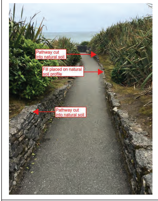
Photograph 3: Observed cut/fill locations at Location 7.
