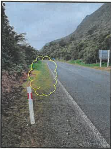
Section 4 2 Looking north along SH6
