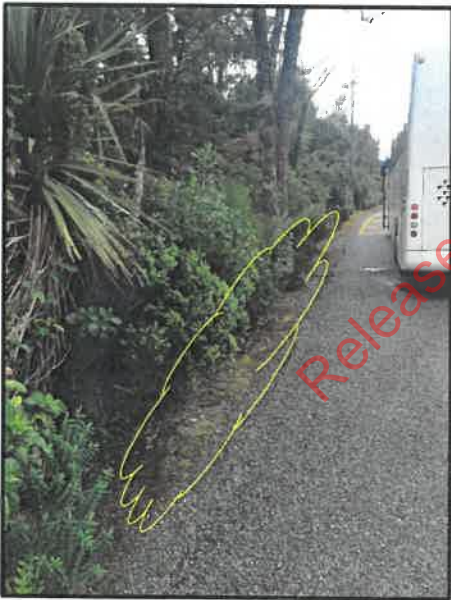
Section 1 4 Looking north behind the bus stop
