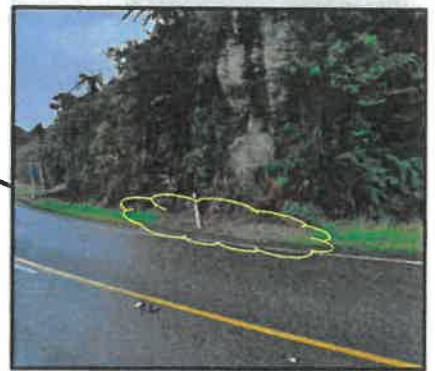
Section 2 2 Looking across SH6 to bluff
