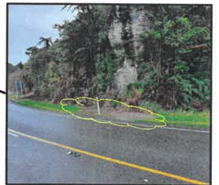
Section 2 2 Looking across SH6 to bluff
