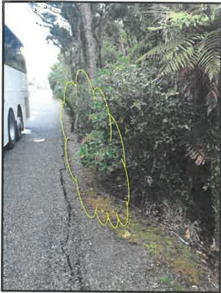
Section 1 3 Looking south behind the bus stop
