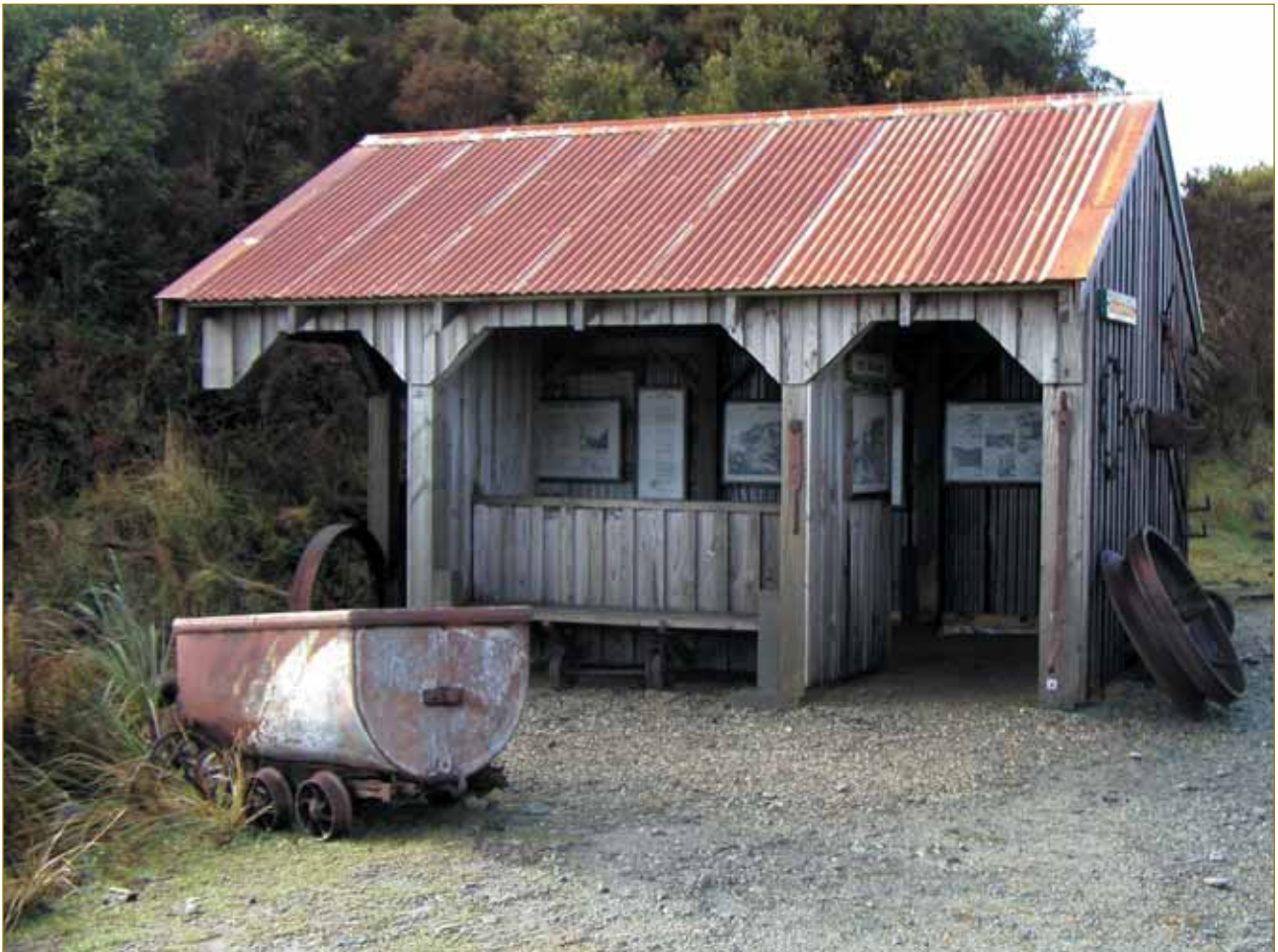
Interpretation shelter at Denniston using recycled materials to emulate a mine shed, and surrounded by mine artefacts. Photo: P.J. Mahoney
