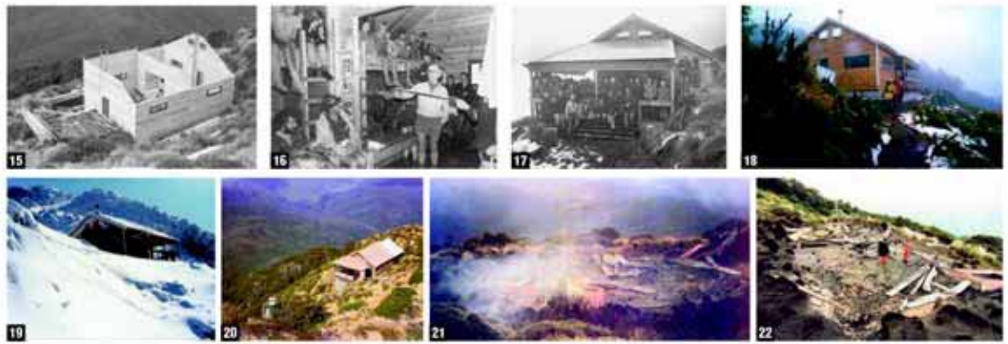
15 Ground hut under construction, 22 March 1981 16 A new construction, oak and pine, built by HVTCT and Forest Service 17 Opening of second Powell Hut, 7 June 1981 18 Windy conditions on opening day, 7 June 1981 19 Hut into the snow 20 Powell Hut under construction and new building, 10 September 1981 21 Smoking system, 17 May 1988 22 Demolition of the hut after the fire, 2009
