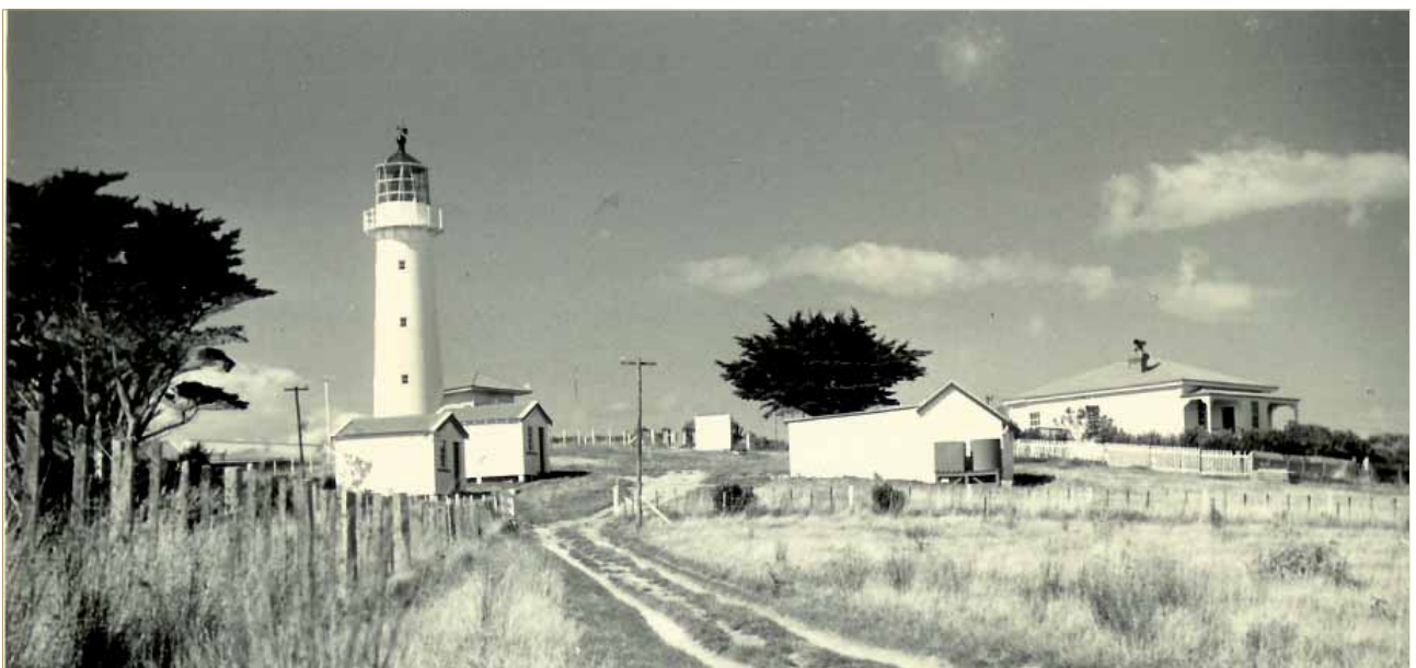
Lighthouse station c.1965. Taylor collection
