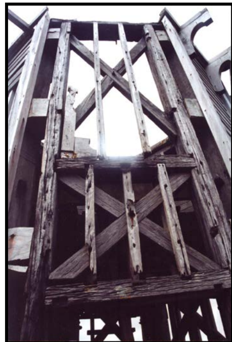
Figure 2: The Lighthouse before the dome was removed in 1939 (left). Figure 3: The ironbark framework before re-cladding in 2001 (right).
