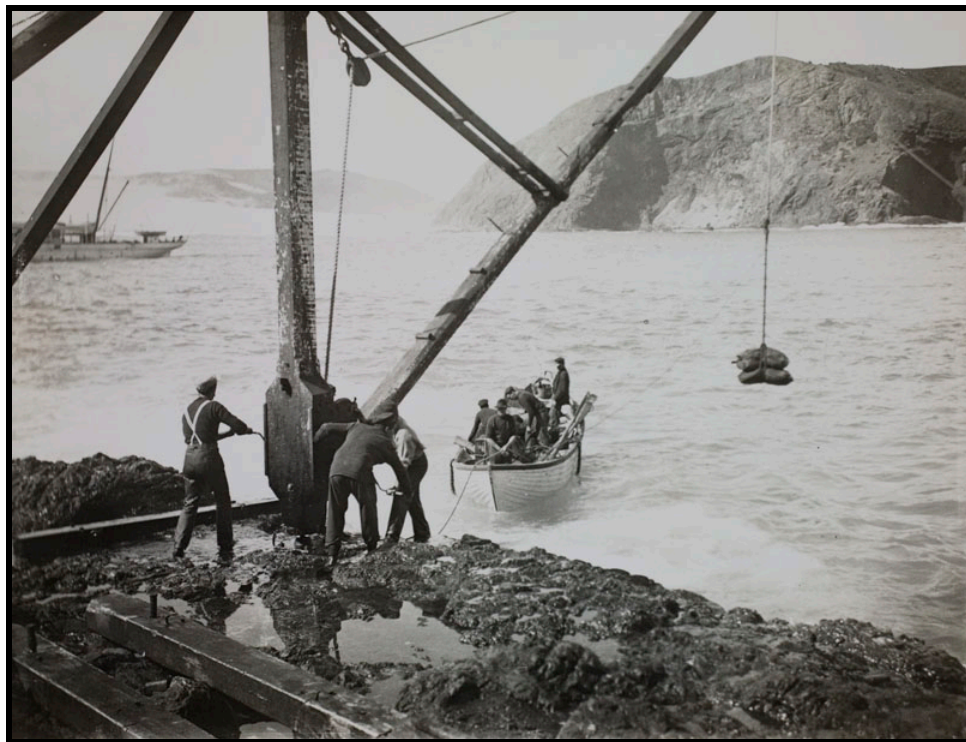
Figure 2: Using a lighter (small boat) to unload from the supply ship (pre 1908) (photo credit: Auckland Museum).
