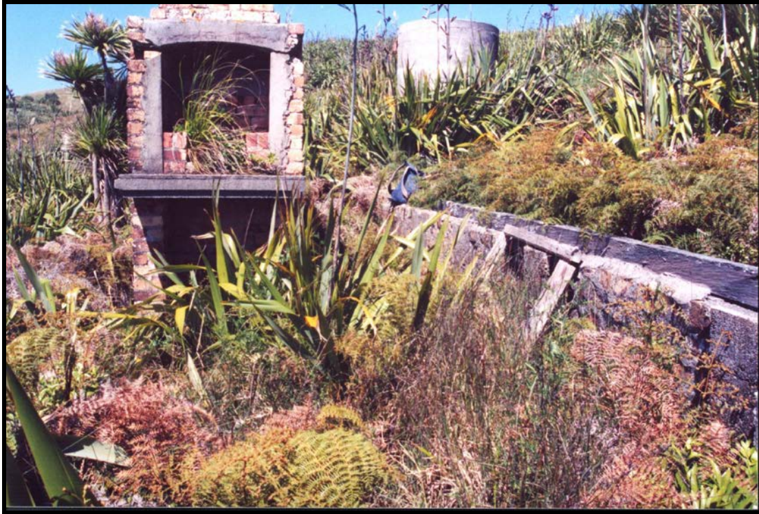
Figure 8: A fireplace, foundations, and water tank at the site of one of the relocated lighthouse keepers houses at the southern end of the island..
