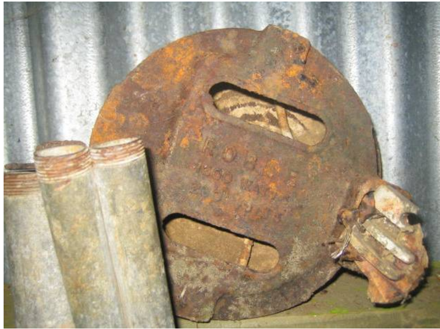
Figure 14: Part of the transformers located in the powerhouse (DoC 2011)
