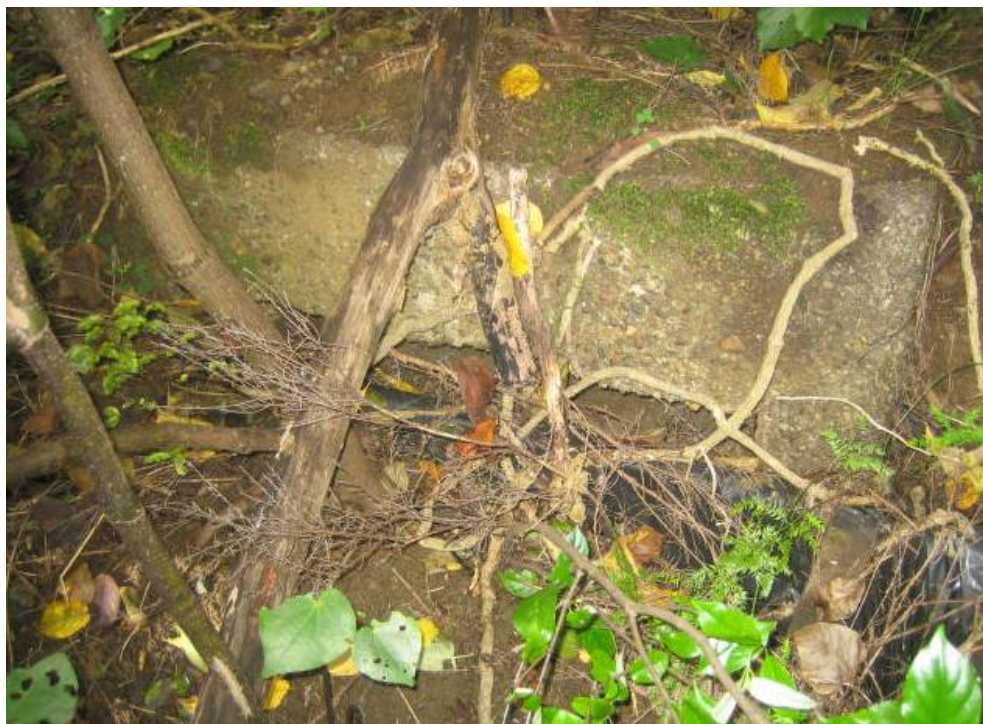
Figure 11: The headgate now filled in (DoC 2011).
