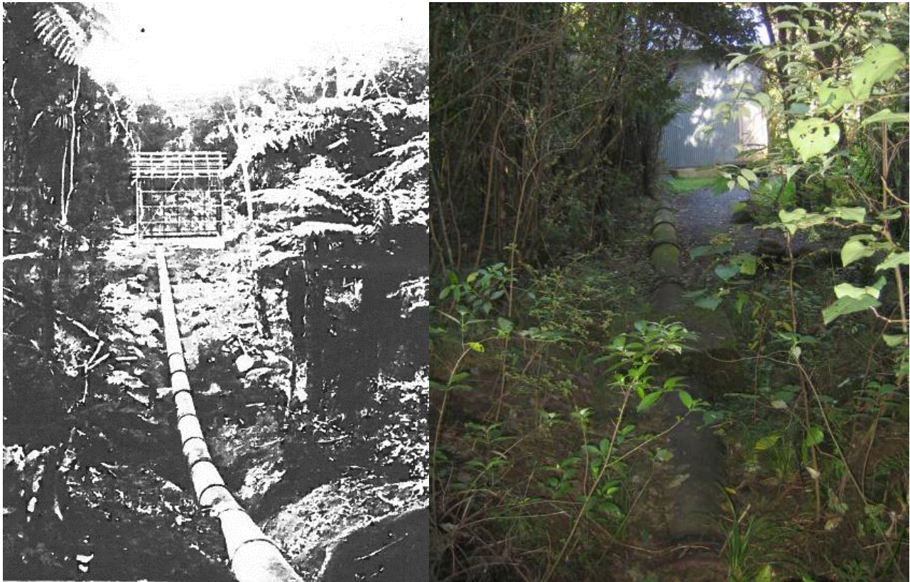
Figure 4: The powerhouse under construction (BOIEPB)
