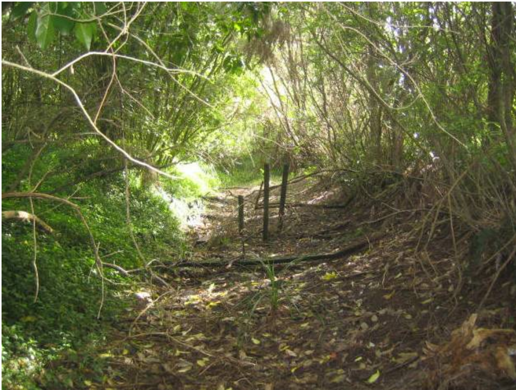
Figure 10: Earth dam. Taken from the headgate forebay that narrows down into the race (DoC 2011)
