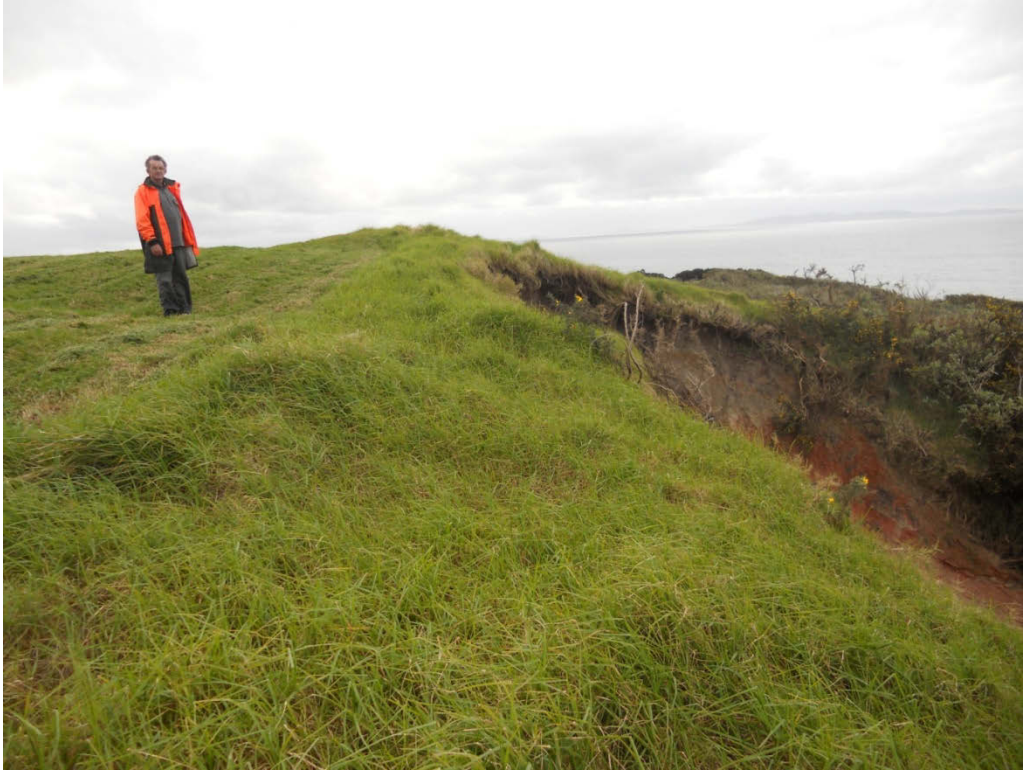
Figure 21: Recent slip on north side of Taumarumaru Pa, and adjacent pits.
