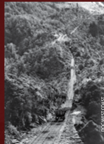
(TOP) BRAKEHEAD VIEW A Q wagon awaits descent at the top of the Incline. The haulage cable used on the Incline was 32mm diameter steel rope.
