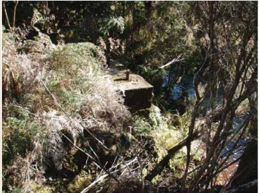
Photo 18: NZFS bridge abutment
