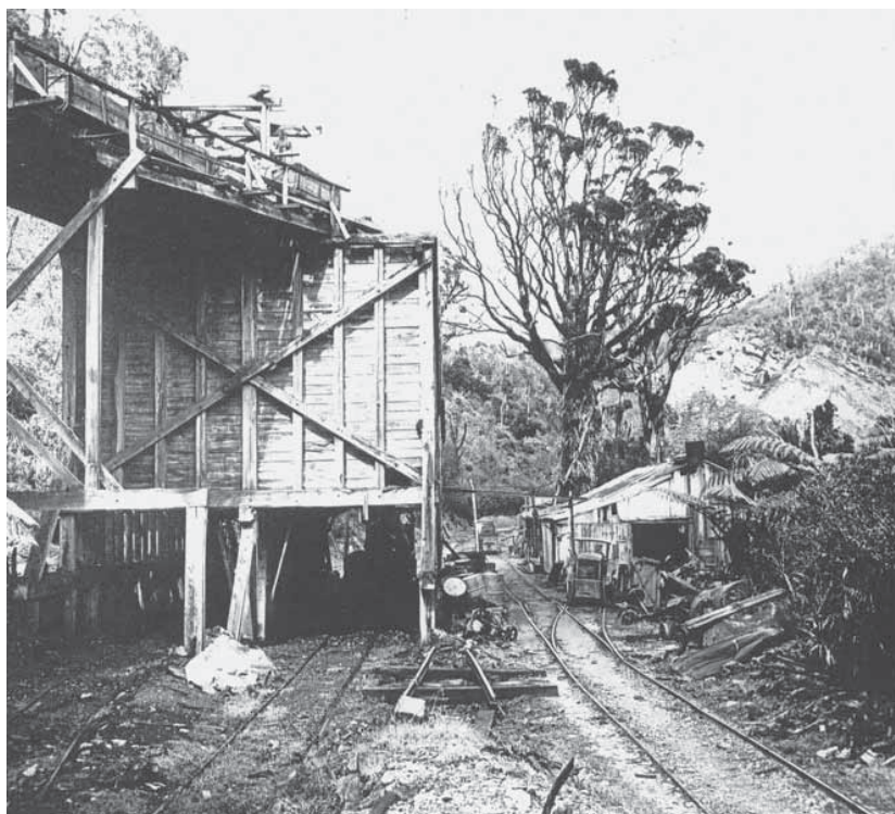
Photo 7: The bins at Ngakawau in 1945, showing coal bins and the high level siding. Note the trestles leading to the tipper at the top of the bins. NZR Q-wagons were shunted underneath the bins for loading and then hauled to the mainline at Ngakawau. The workshop is to the right. ATL PASCOE COLLN 1356%, WAR EFFORT COLLECTION
