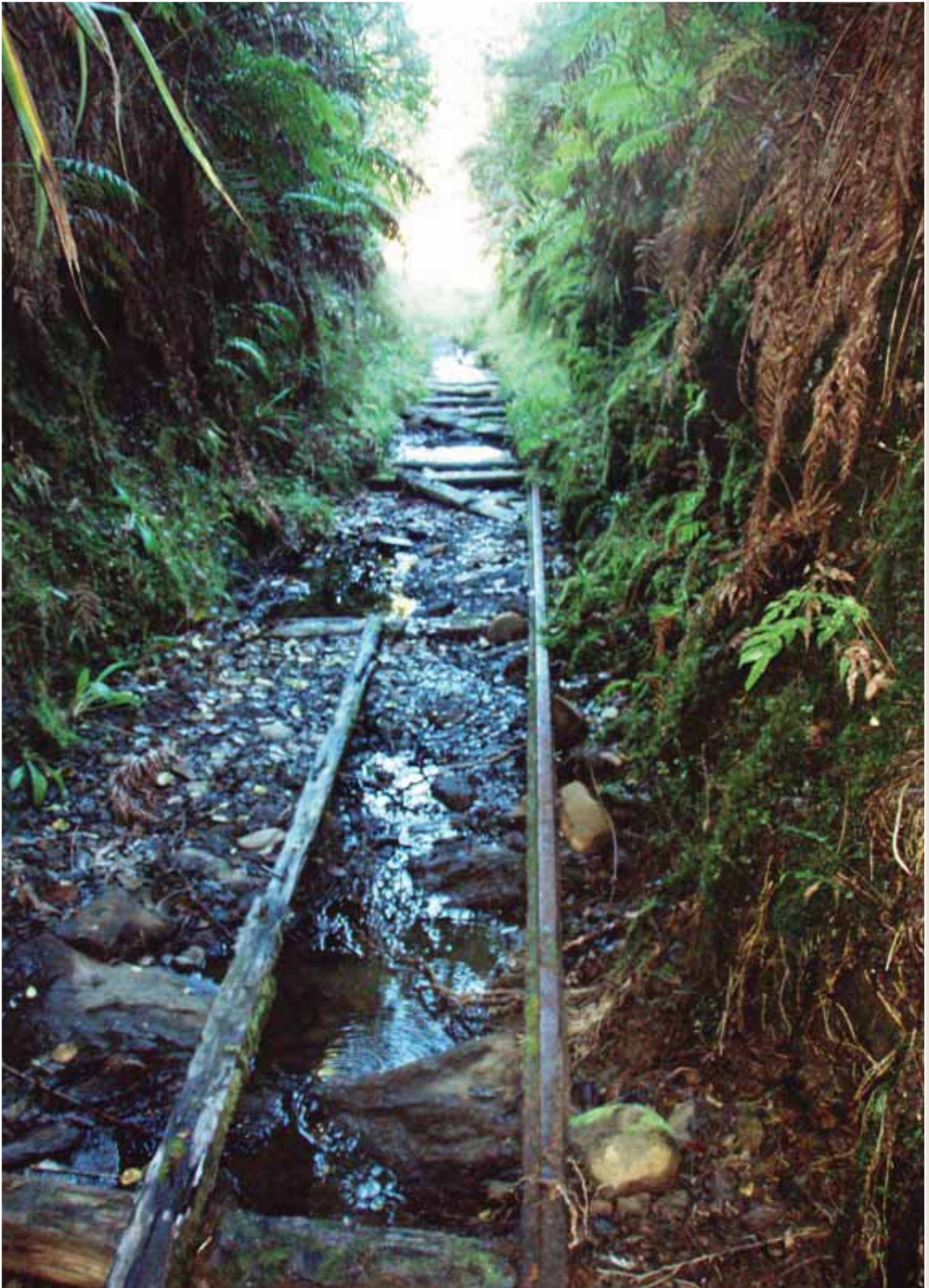
Photo 21: Looking west from Papa Tunnel entrance.
