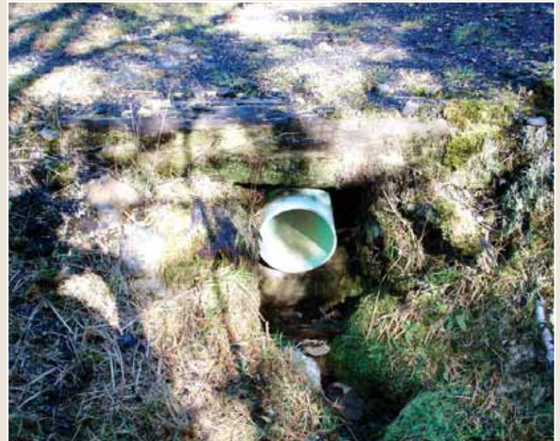
Photo 44: Old pig sty culvert with modern culvert inside it.
