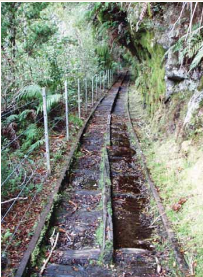
Photos 63 and 64: Centre rail brake at the southern end of The Veranda and the north side of the Mangatini Tunnel.
