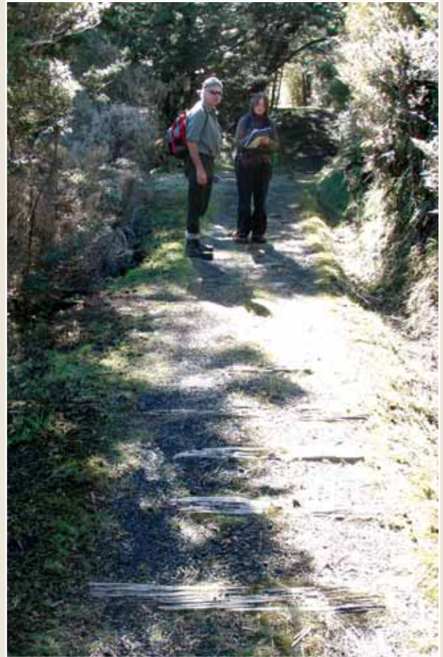
Photo 40: Section of tramway showing sleepers
