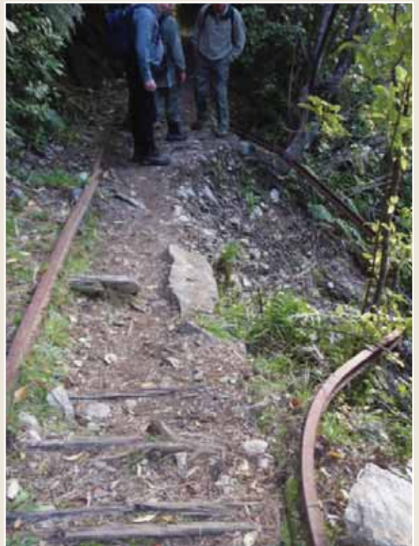
Photos 78 and 79: Two sections of damaged tramway caused by rock falls.
