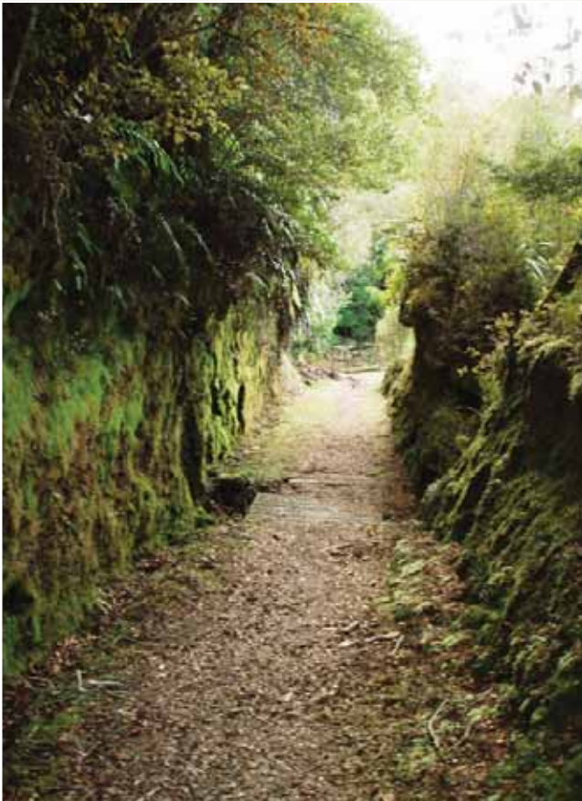
Photo 54: Right - Cutting with side drain.
