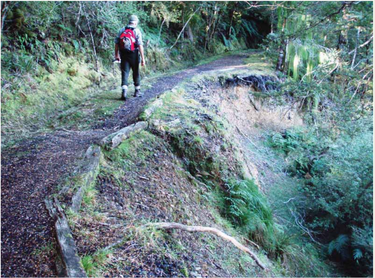
Photo 42: Edge of tramway showing a large area slumped away.
