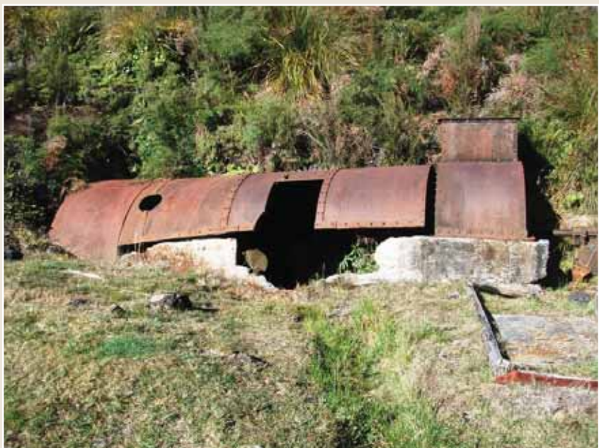
Photo 14: Fan house at the mine.
