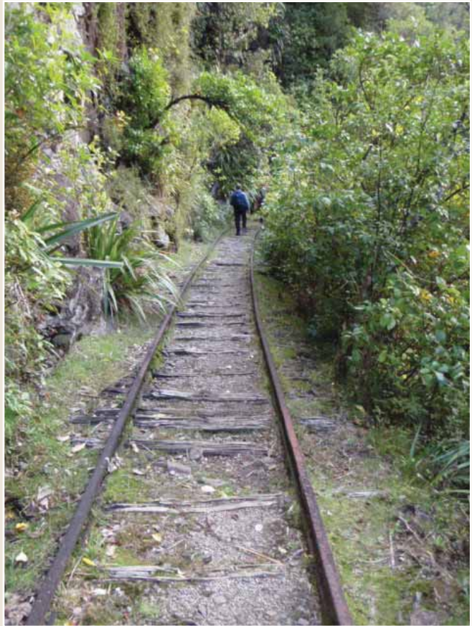
Photo 74: A good section of alignment, typical of the more intact parts of this section. N. COOKE 2008
