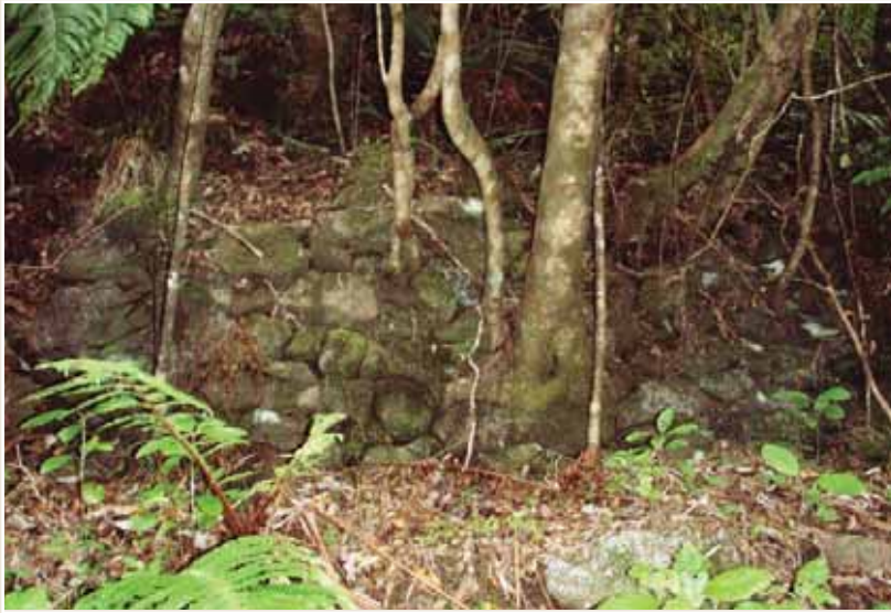
Photo 76: Hand stacked rock wall.
