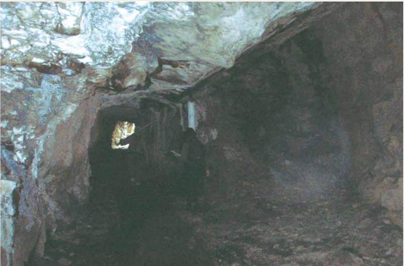
Photo 75: Irishman's Tunnel. The large excavation on the right is an alignment mistake made during the creation of the tunnel.
