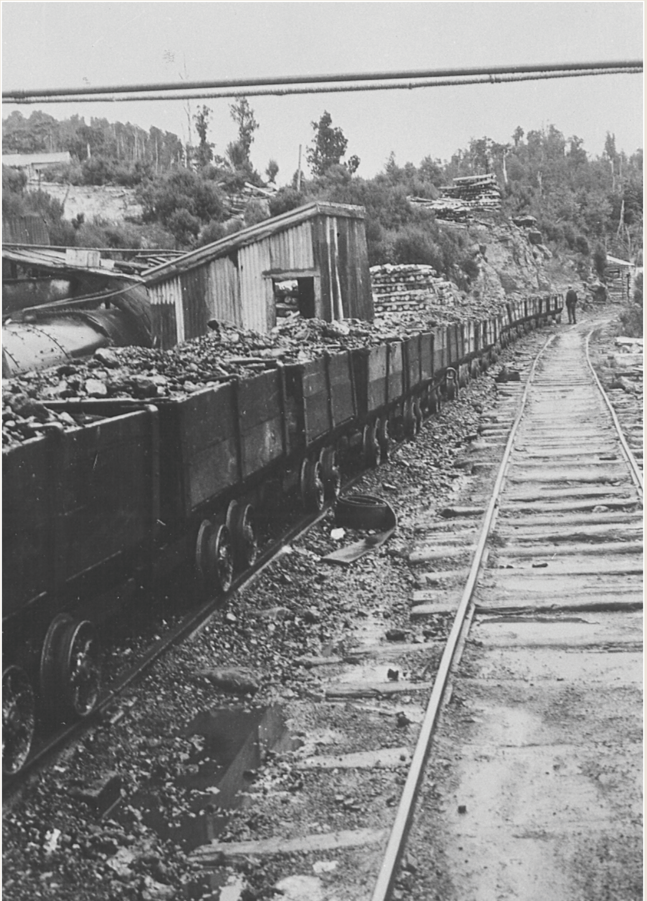
Photo 15: 1940s tramline view. The fanhouse and associated building are seen on the right of the image. Note the double track of tram, with the right hand line being slightly higher than the left.
