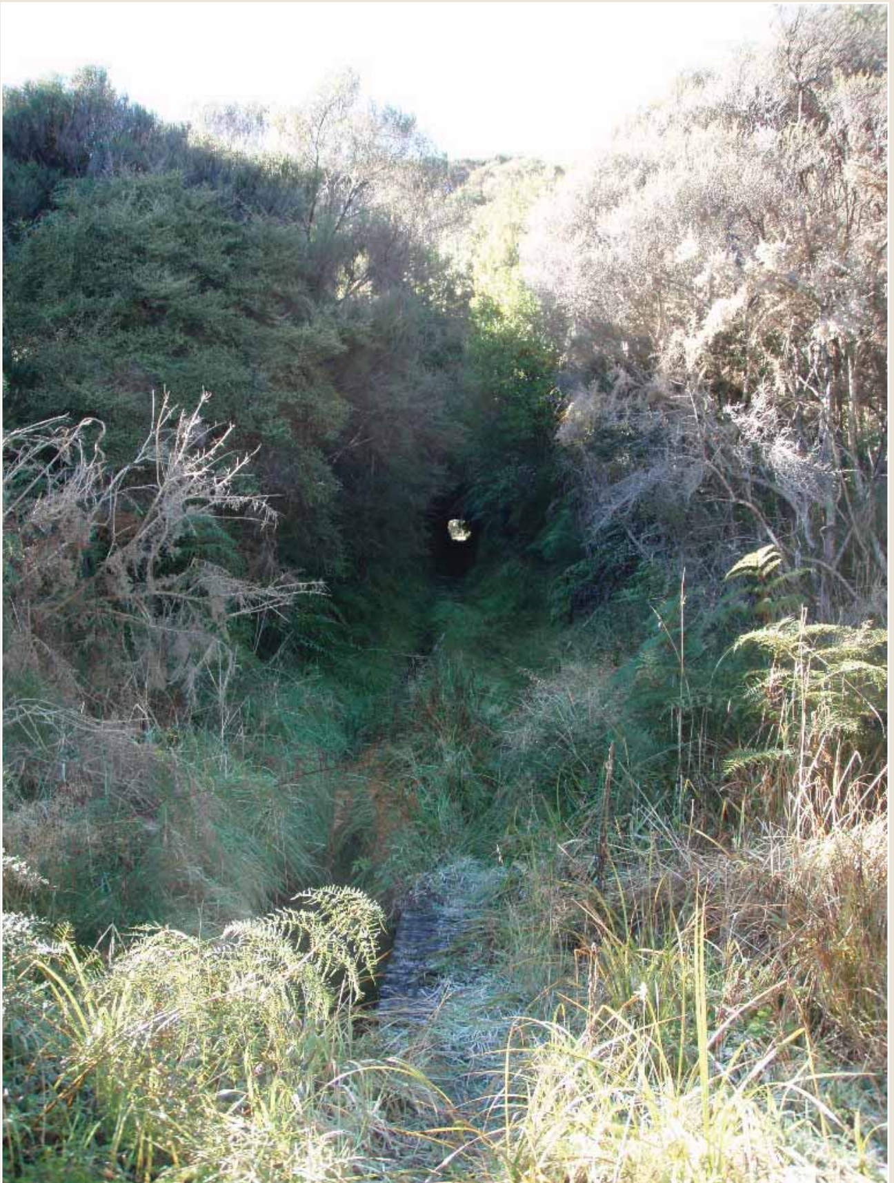
Photo 23: Looking east towards Papa Tunnel. Note the encroaching vegetation.
