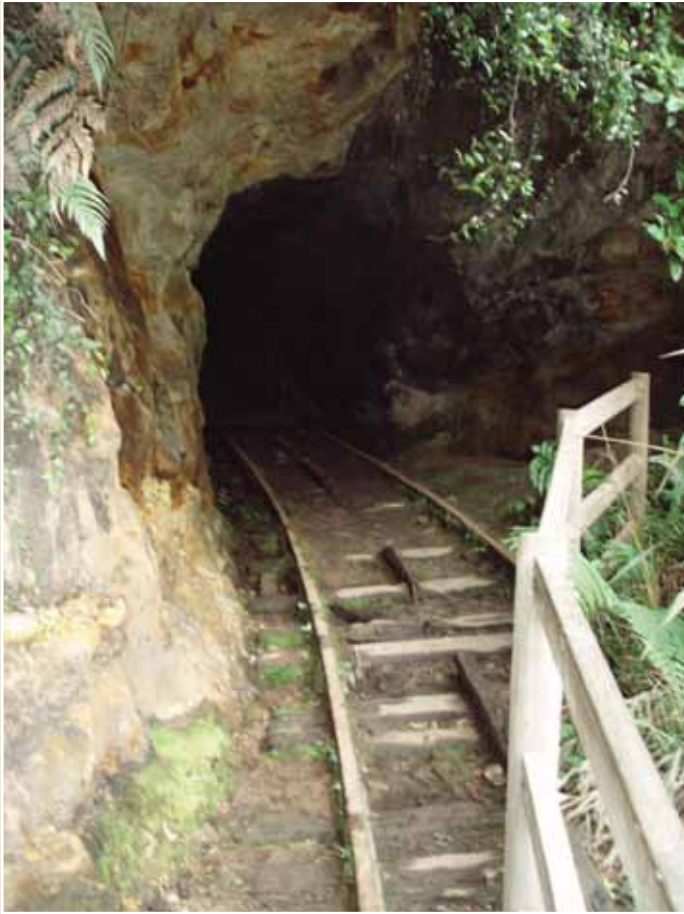
Photo 68: Western end of the Mangatini tunnel where it comes out into the Ngakawau gorge.
