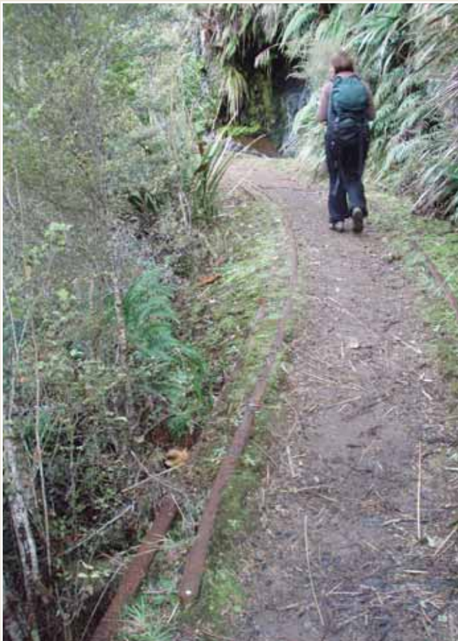
Photo 61: Section of in situ rail. Note the check rail bottom left. An extra safety measure to keep the tram on the rails as it negotiated tight corners.
