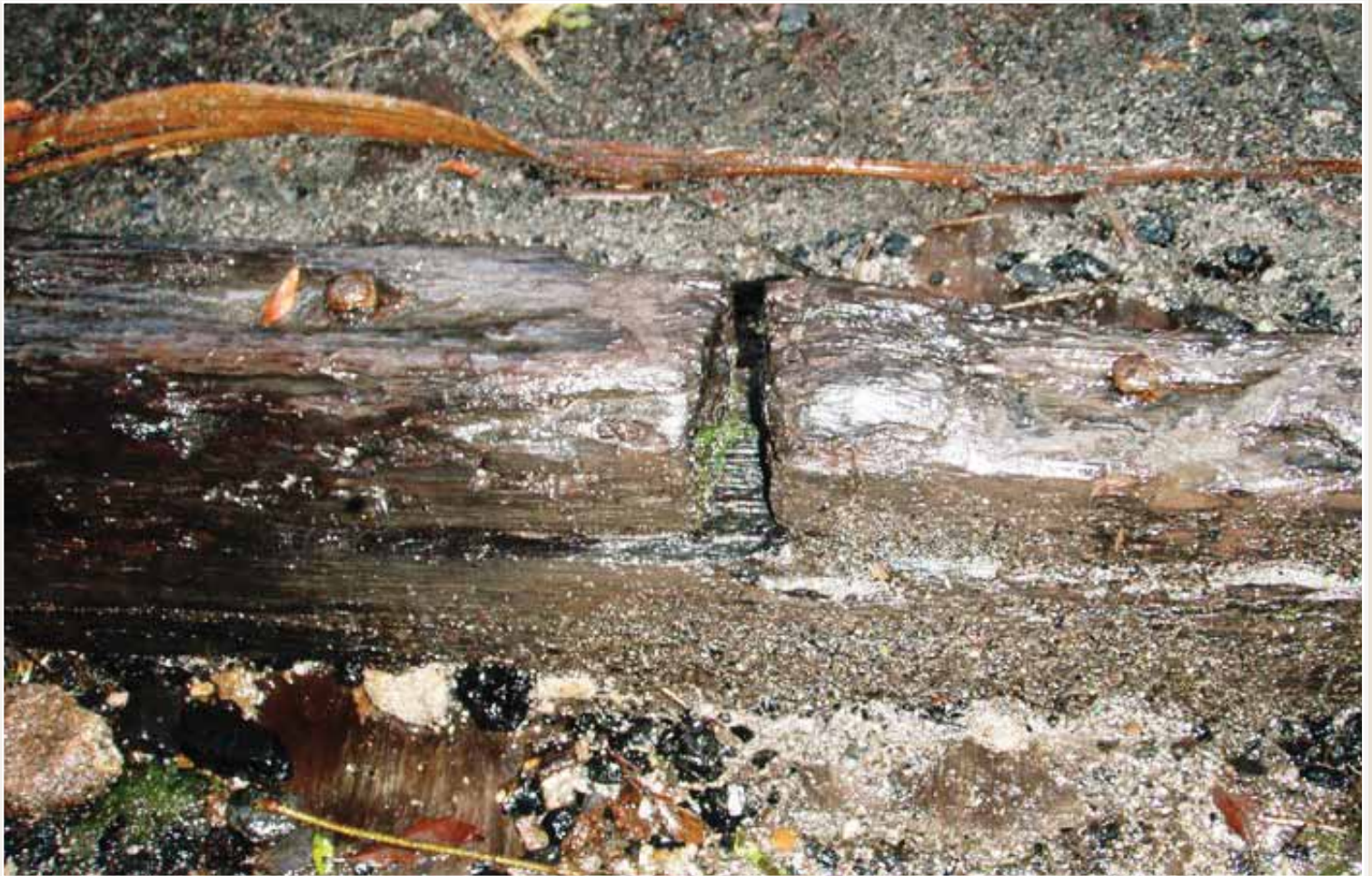
Photo 65: Detail side view of centre rail brake showing the placement of timbers
