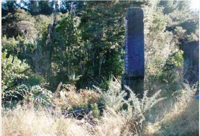
Photo 13: Chimney on the mine office and storeroom site.
