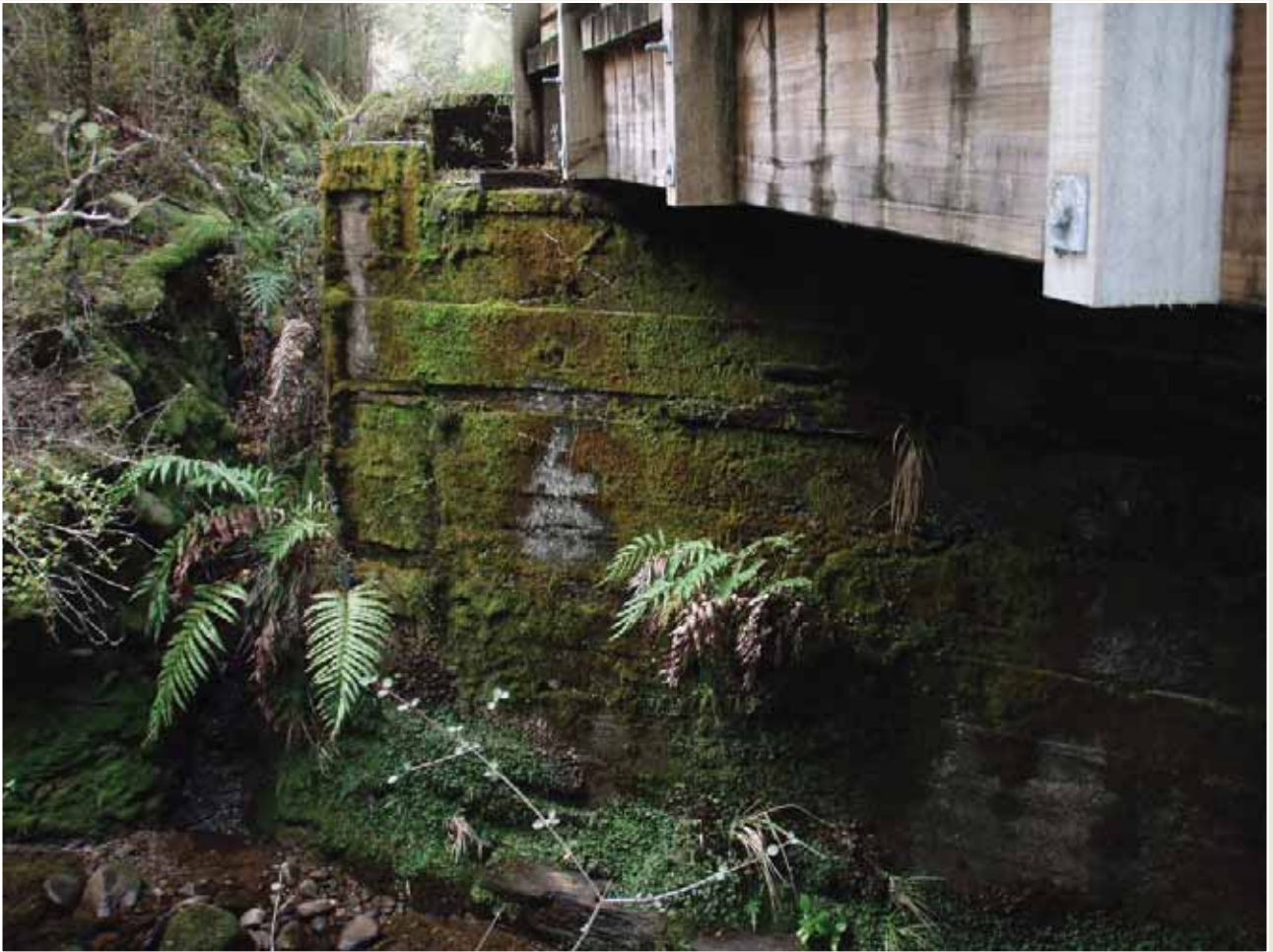
Photo 51: Modern bridge built on old concrete abutments.
