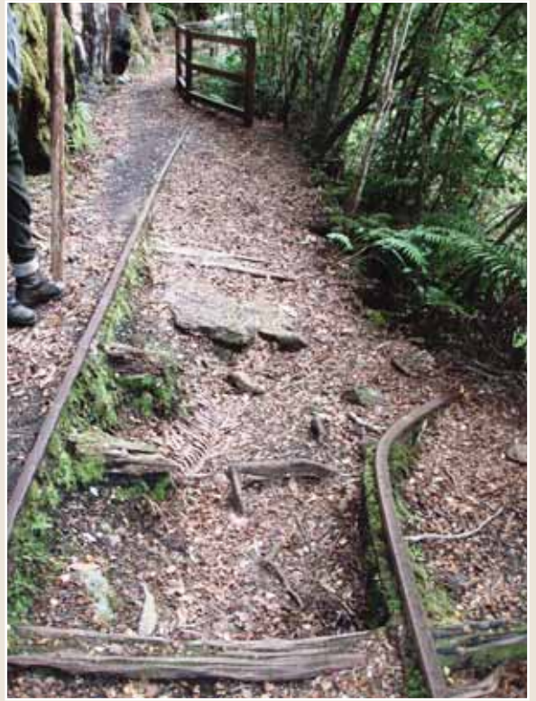
Photos 78 and 79: Two sections of damaged tramway caused by rock falls.
