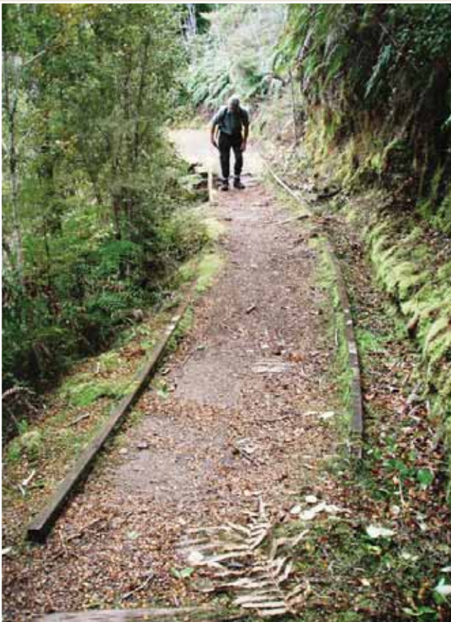
Photo 52: In-situ rail on a side benched formation.
