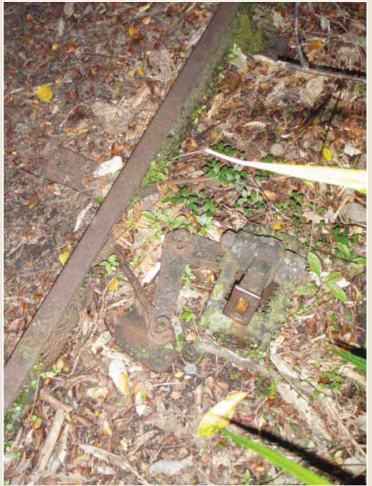
Photo 84: Part of a points lever mechanism. N. COOKE, 2008
