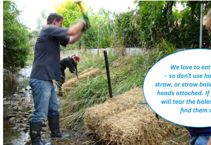
Securing the straw bales in place.
