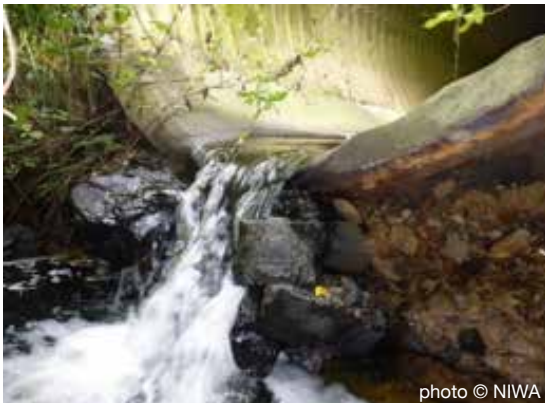
FIGURE 3: Perched culvert in the lower reaches of Martin Stream under Hakarimata Road
