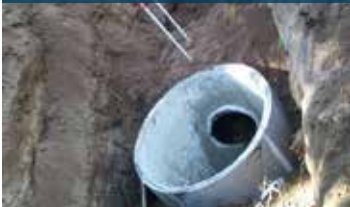
'Kōkopu Condo' under construction. The white rods with red tape are attached to antennae installed to detect condo use by fish implanted with Passive Integrated Transponder (PIT) tags.
