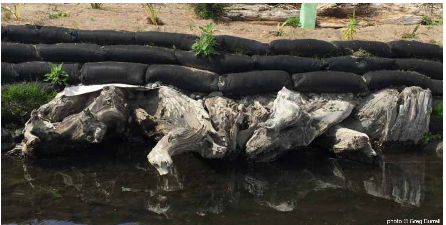
FIGURE 6: A wood fish refuge incorporated into the bank of Kaputone/Kā Pūtahi Creek to provide fish cover.
