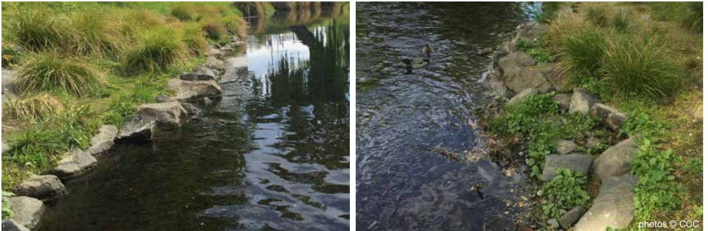
FIGURE 5: Boulders placed along the water edge to provide fish habitat in a Christchurch urban river. In both photographs, an alcove has been created to enhance habitat, but sediment has accumulated in the alcove on the right, due to a backwatering effect.
