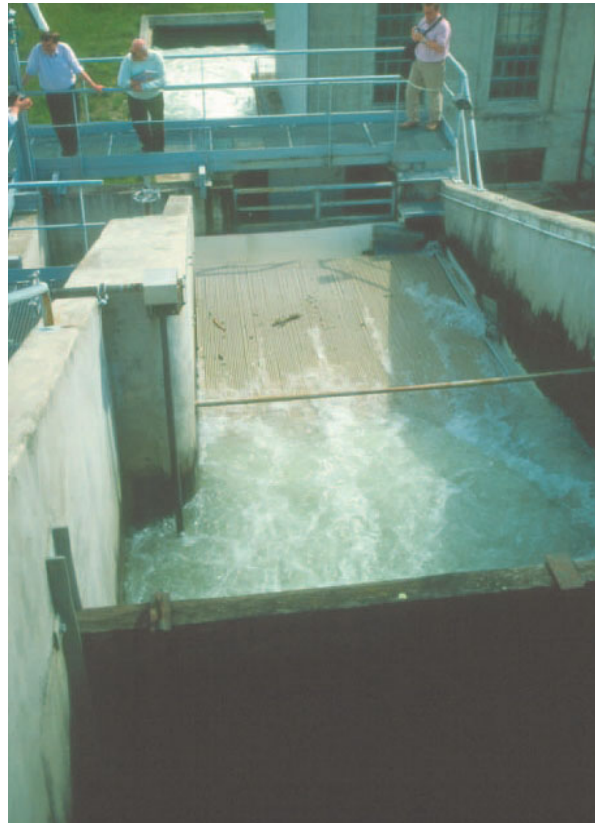
Figure 5.116: Detail of figure 5.115: The bypass water is led to a Tyrolean weir, where a by- pass channel is installed at the downstream end, which receives fish and guides them into a holding pool.
