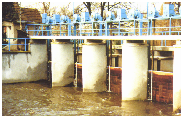
Figure 3.5: Sliding-Panel Weir Egelin on the Bode river (Saxony-Anhalt)
