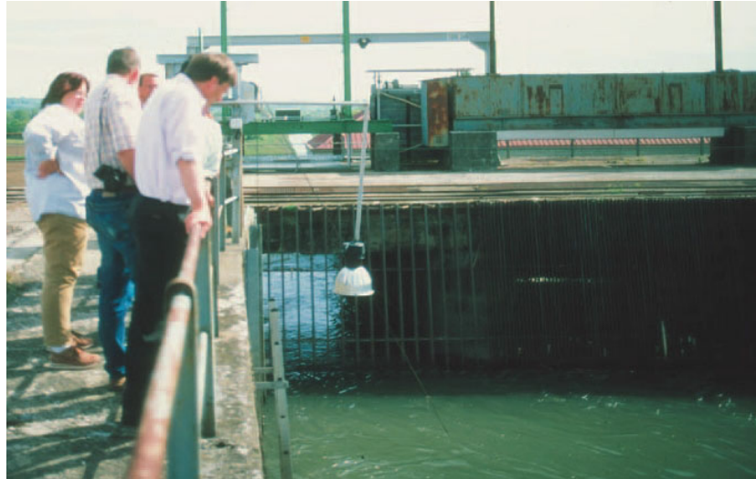
Figure 5.114: Bypass at the side of the screen of the hydropower plant Camon (Garonne / France)
