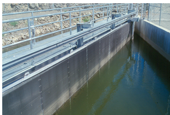
Figure 5.83: Detailed view of figure 5.82: A brush-system is operated horizontally over the perforated plate screen. The bypass inlet can be seen on the right hand side of the picture.
