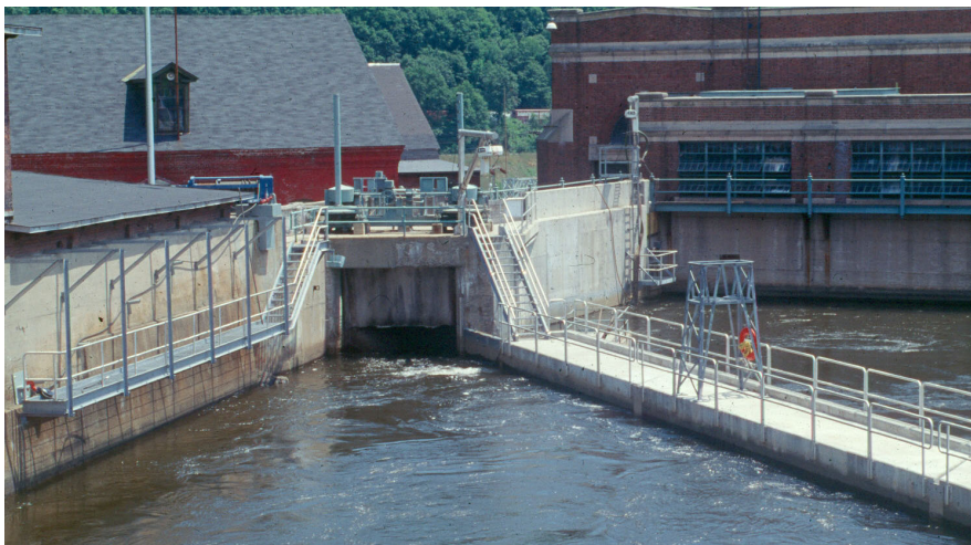
Figure 5.81: Detailed view of figure 5.80: Intake of bypass with actuation to adjust the overflow height
