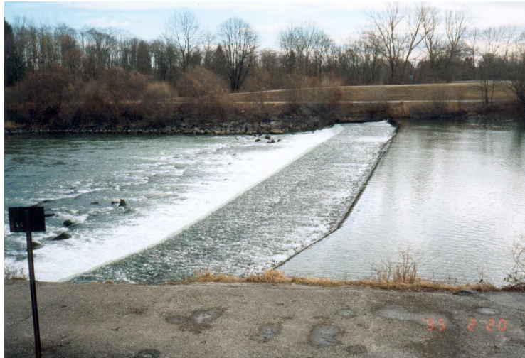
Figure 3.3: Stepped Drop on the Lech river south of Augsburg (Bavaria)
