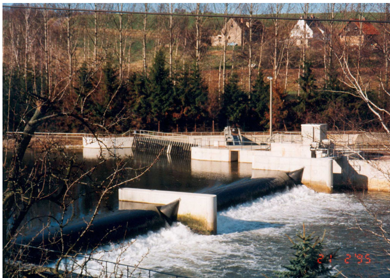
Figure 3.12: Inflatable weir Thierbach on the Zwickauer Mulde (Saxony)
