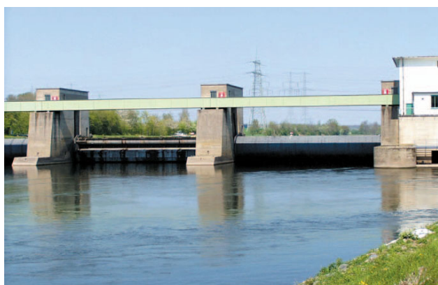
Figure 3.7: Drum gates are installed in the outer fields of the weir of the Main barrage Garstadt (Bavaria), in the centre field a gate on which a gate is placed
