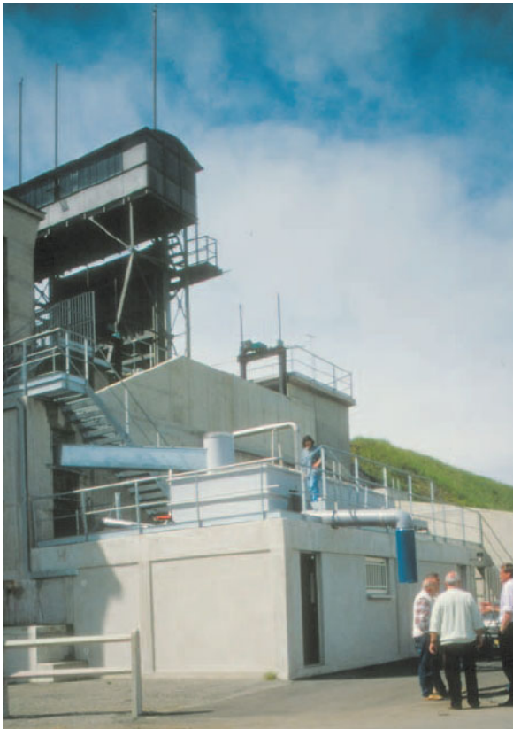
Figure 5.115: Total view of the trapping system for downstream mi-grating smolts at the weir Pointis (Garonne / France)
