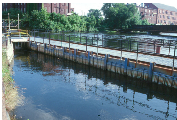
Figure 5.75: Louver in the headwater channel of the Holyoke Dam on the Connecticut river (Massachusetts, USA).
