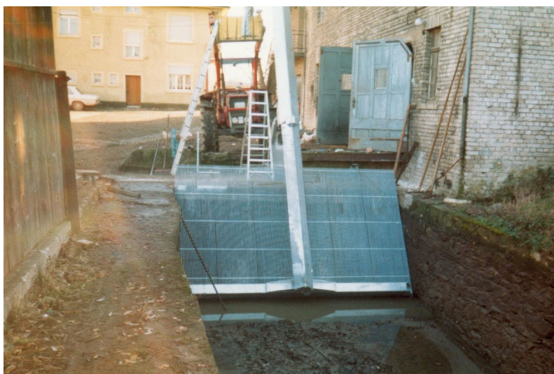
Figure 5.31: Screen with hydraulic screen cleaning machine in a small discharging power plant on the Dill river (Hesse, Germany)
