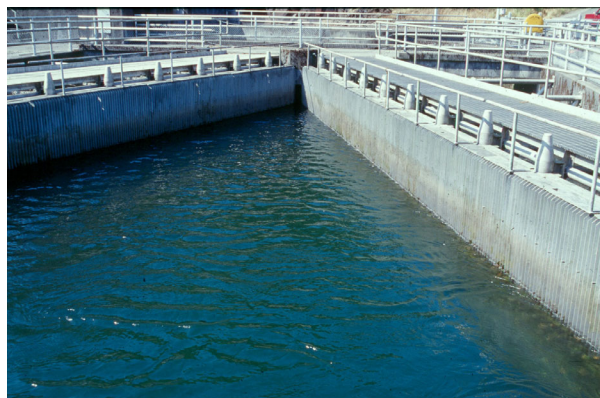
Figure 5.93: Louver for Pacific salmonids with a bypass arranged in the centre (Collwitz Falls, Washington State, USA)
