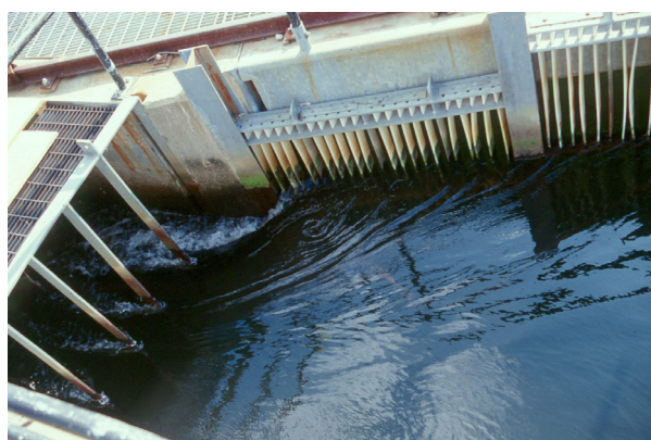
Figure 5.76: Detailed view of figure 5.75: Intake of bypass
