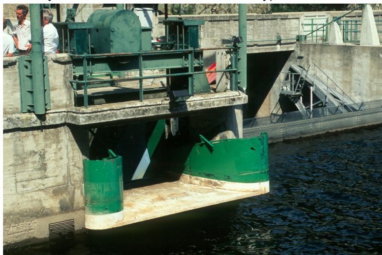
Figure 5.68: The bypass can be adjusted in height and thus aligned to changing levels of the headwater. It can also be hoisted above the water surface outside the migration sea-season of salmon smolts
