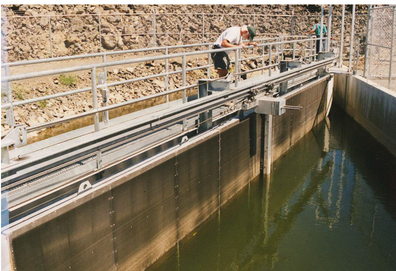
Figure 5.39: Stationary screens with perforated plate ( d = 3.0 mm) at a withdrawal point for irrigation purposes in the catchment area of the Yakima River (Washington State, USA)
