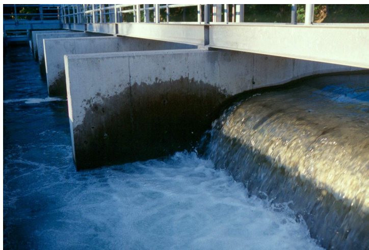
Figure 5.112: Overflow weir with integrated Wedge-Wire-Screen at an intake for an irrigation channel (Oregon, USA)
