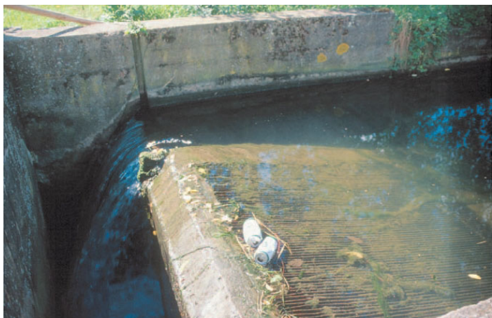
Figure 5.107: Flat screen of the Klostermuehle (mill) in the Solz river (Hesse, Germany) with an inclination of \alpha < 45^\circ and a clear width of 20 mm
