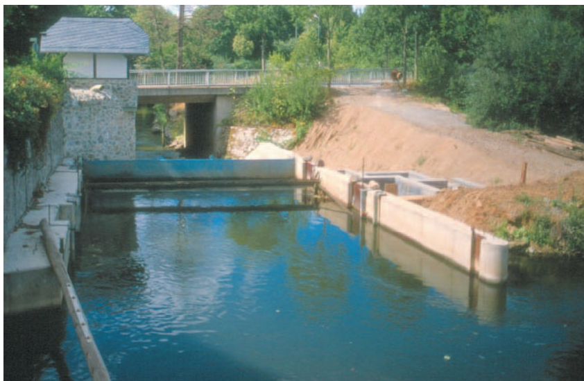
Figure 5.40: Overflowable hydropower plant at the Lahn river in Wetzlar (Hesse, Germany) with a flat inclined 10 mm-perforated plate screen
