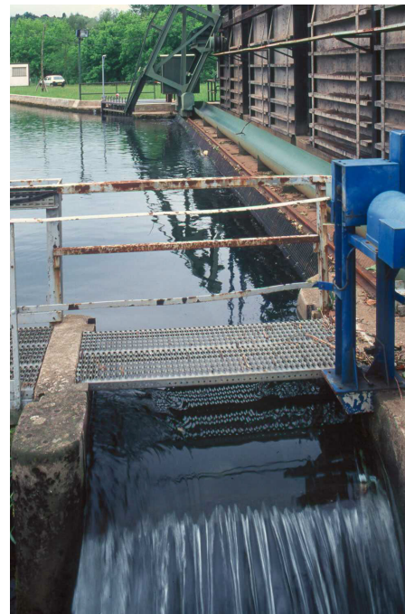
Figure 5.74: The bypass at the power plant Halsou (Nive river, France) directly joins the intake screen that is approached by the flow tangentially
