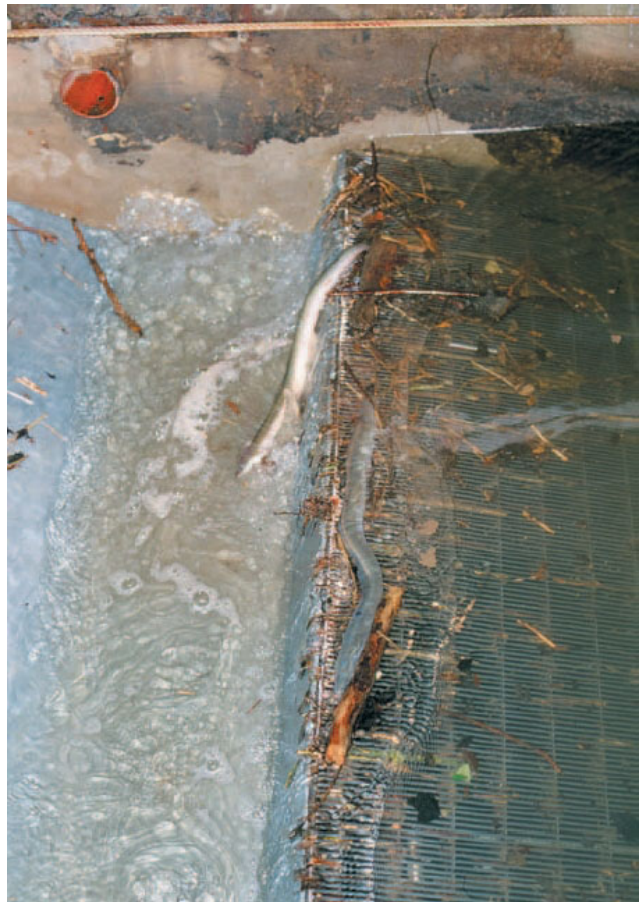
Figure 5.110: Eel which are passing the top edge of the flat screen at the Floecksmuehle (mill) in the Nette river (Rhineland-Palatinate) and then reach the traversing bypass channel
