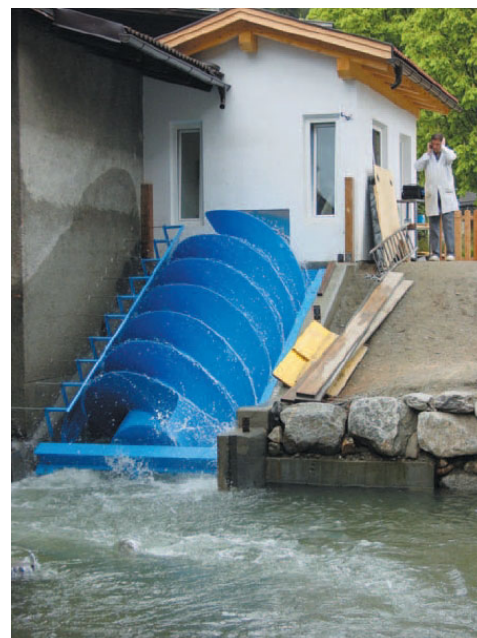
Figure 3.24: Archimedean screw with a capacity of 20.5 kW at a head of 2.0 m and an design flow of 1.2 m 3 /s (mills in Taufers/South Tyrol)
