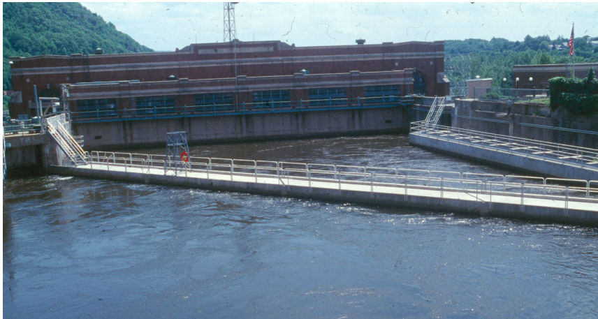
Figure 5.80: The skimming wall at the hydropower plant Bellows Falls on the Connecticut river (Connecticut, USA) has an immersion depth of 4.6 m. The bypass opening can be seen on the left hand side of the picture
