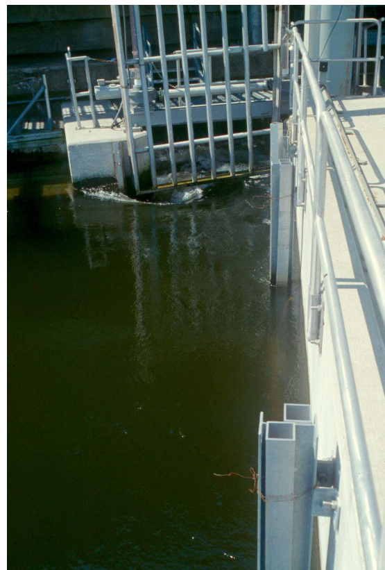
Figure 5.78: Louver at the hydropower plant Vernon Dam on the Connecticut river (Connecticut, USA) with a view towards the bypass: The visible coarse screen initially caused shunning and avoidance reactions of downstream migrating smolts when the operation was started. It has meanwhile been removed
