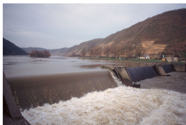
Figure 3.8: Drum gate of the Moselle barrage Lehmen (Rhineland-Palatina)
