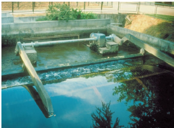
Figure 5.108: Flat screen with a traversing bypass channel at a hydropower plant in the Allier river near Langeac (France), which has proven less effective because of a too large clear width
