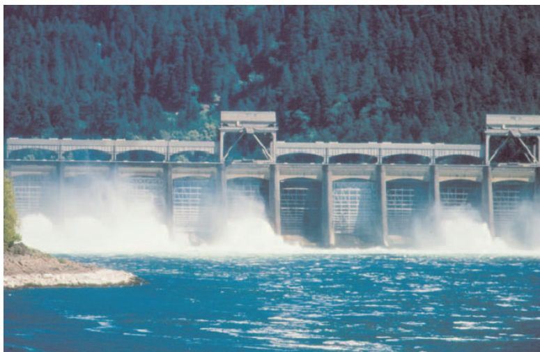
Figure 4.1: Dispersion of the weir structure through a ski jump-like design of the sluices at the Bonneville Dam (Columbia River, USA) for the purpose of reducing the mortality of migrating smolts of salmonids
