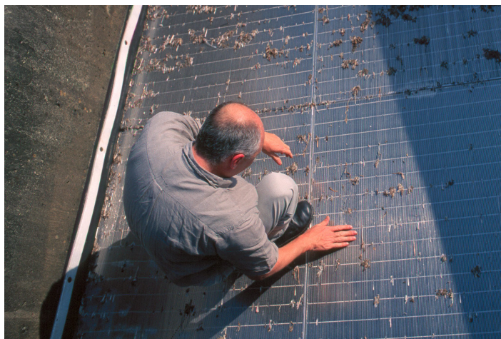
Figure 6.11: Detail of figure 6.10: The very small bar spacing of 1 mm of the flat inclined Wedge-Wire-Screen and the very smooth surface minimize the risk of injuries for fish
