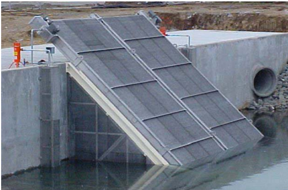
Plate 3.10 Example of a self-cleaning belt screen installation. The screens are sealed at the sides to prevent fish or debris entrainment; screened weed and other debris are dumped on the ground below the top of the screen (courtesy of FPI Water Screens, USA: www.fpi-co.com )
