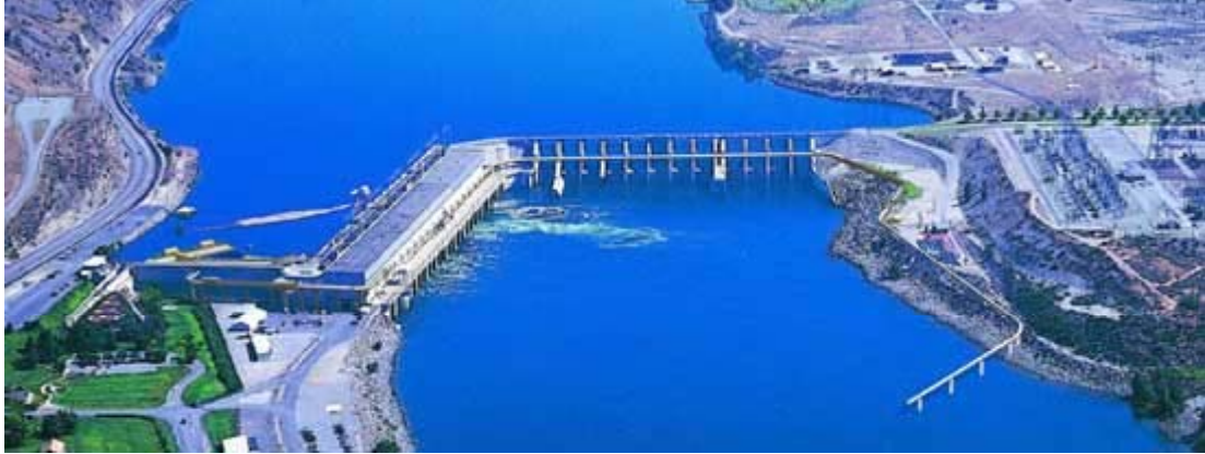
Plate 3.14 Rocky Reach dam with the powerhouse on the left and the bypass pipe in the bottom right (Chelan County PUD).
