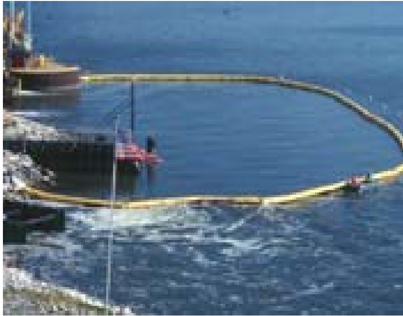
Plate 3.9 Gunderboom MLES barrier in place around an intake structure. The yellow support collar is visible and air backwashing is taking place along part of the barrier.
