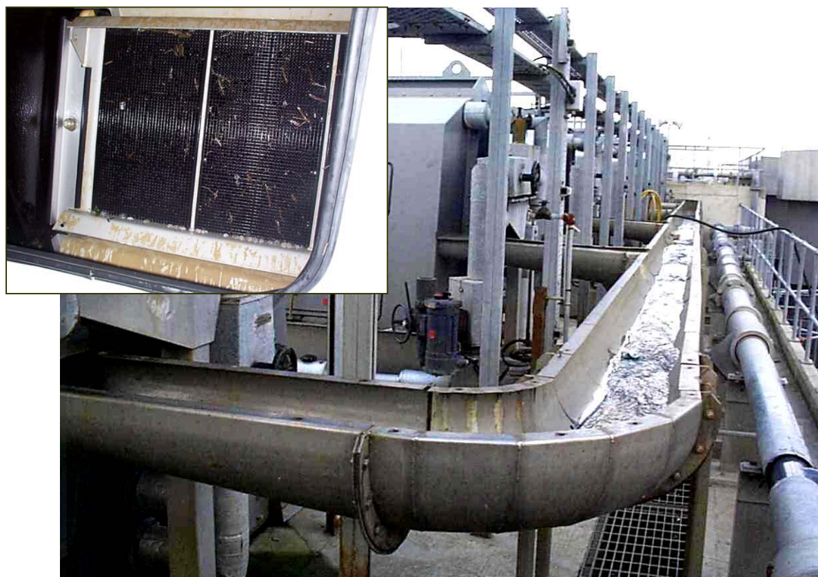
Plate 3.7 Fish Return System at Barking Power Station, Thames Tideway. Insert shows screen panel with fish buckets inverted.
