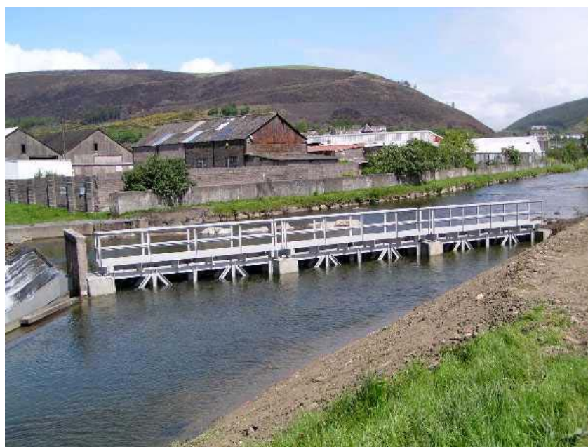
Plate 3.1 Fixed panel screen installed on the R. Afan, Port Talbot in 2003, to prevent salmonid smolts from entering the docks feeder.
