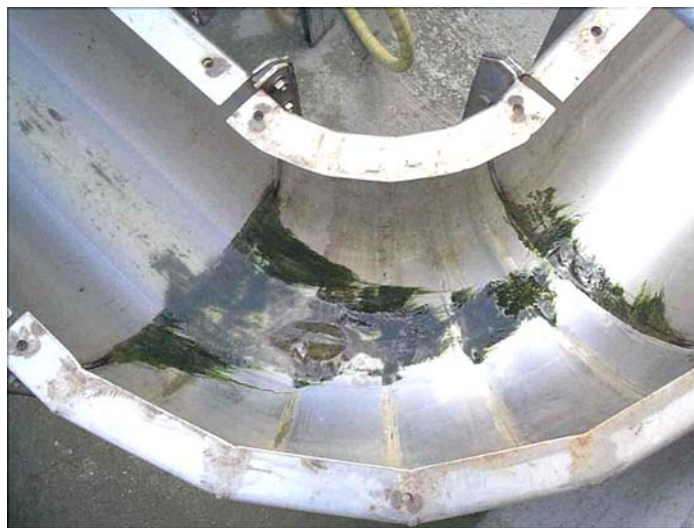
Plate 3.8 A sharp bend in this fish return gully demonstrates the issue of biofouling where uneven joints have encouraged algal growth, causing a flatfish to take cover there. A smooth surface or exclusion of light would have prevented this.
