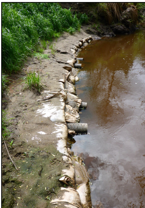
“Tuna townhouse” 150mm flexible pipe in u-shaped lengths set in stream bank was simple and cheap
