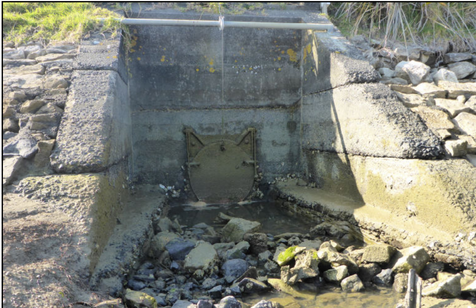
LOW TIDE: meagre low flow with poor/nil connection to water line
