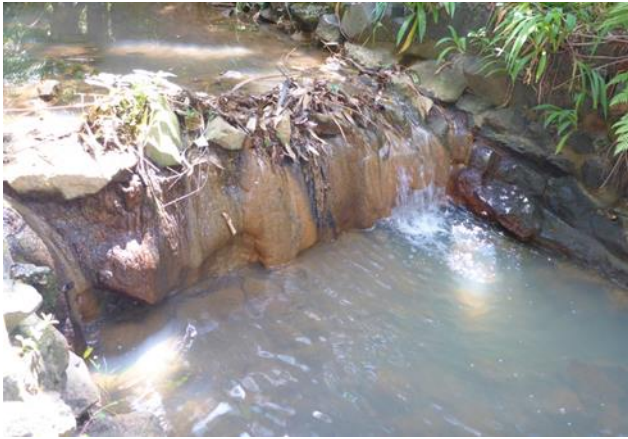
Figure 1: One of four weirs on Gibbons Creek that impeded passage for weak swimming fish, December 2015. Photo: NIWA
