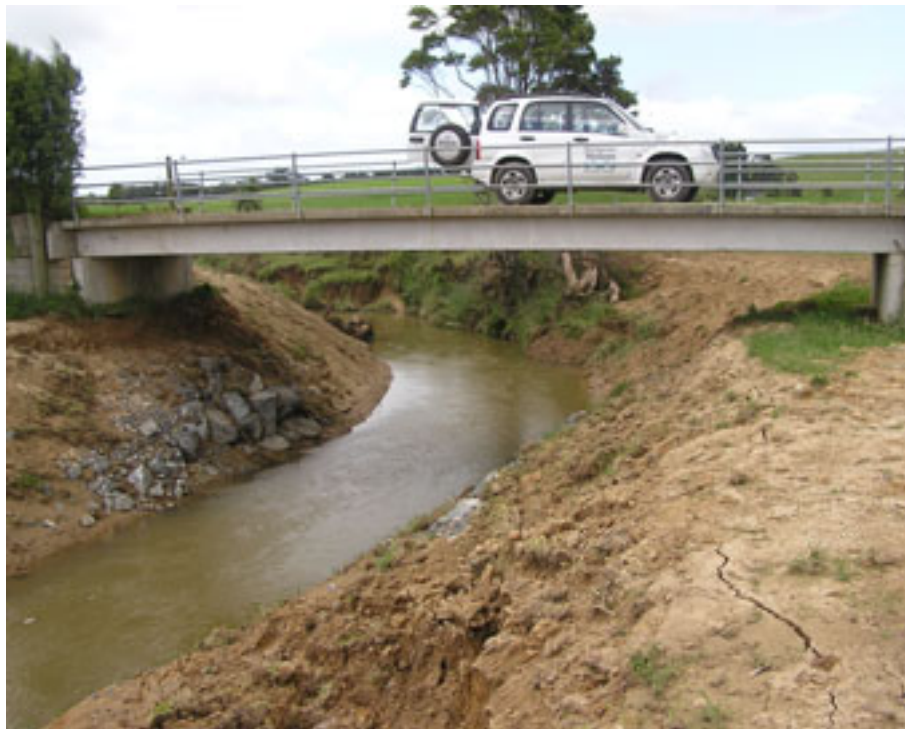
Figure 15 Typical single span farm bridge
