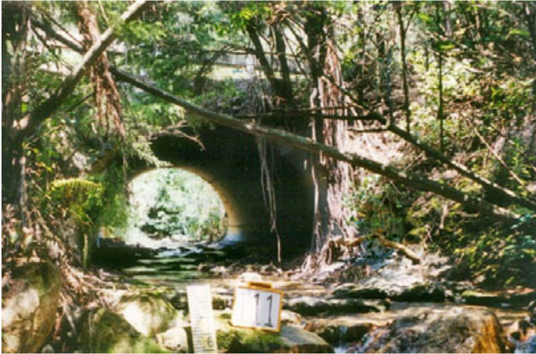
Figure 2 Single barrel arch culvert
