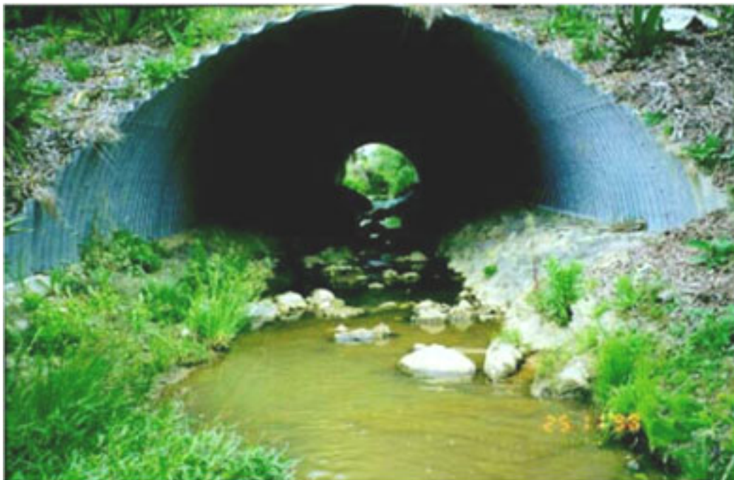
Figure 3 Best Practice - single barrel arch culvert
