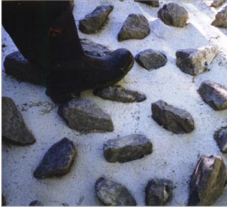
Figure 11 Rocks can be cemented into the base of waterway crossings and/or to the aprons of culverts to ensure that there are areas of low water velocity available to aid fish passage and sediment which is appropriate for invertebrates is retained within the structure
