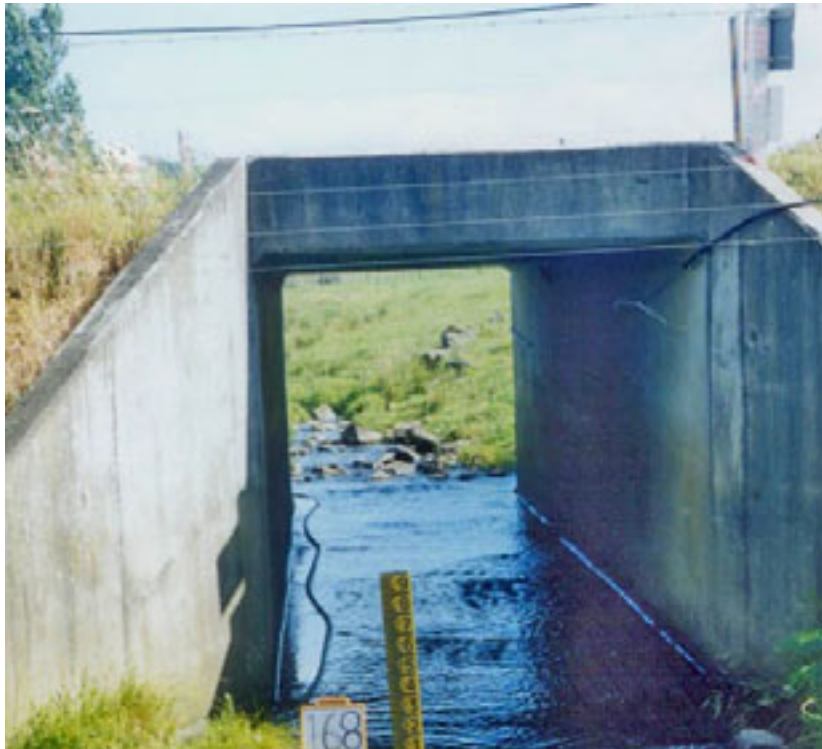
Figure 9 Single box culvert
