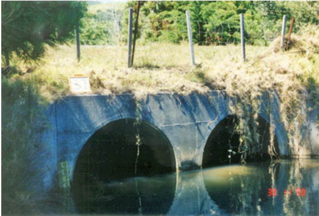
Figure 7 Typical multi-barrel circular culvert
