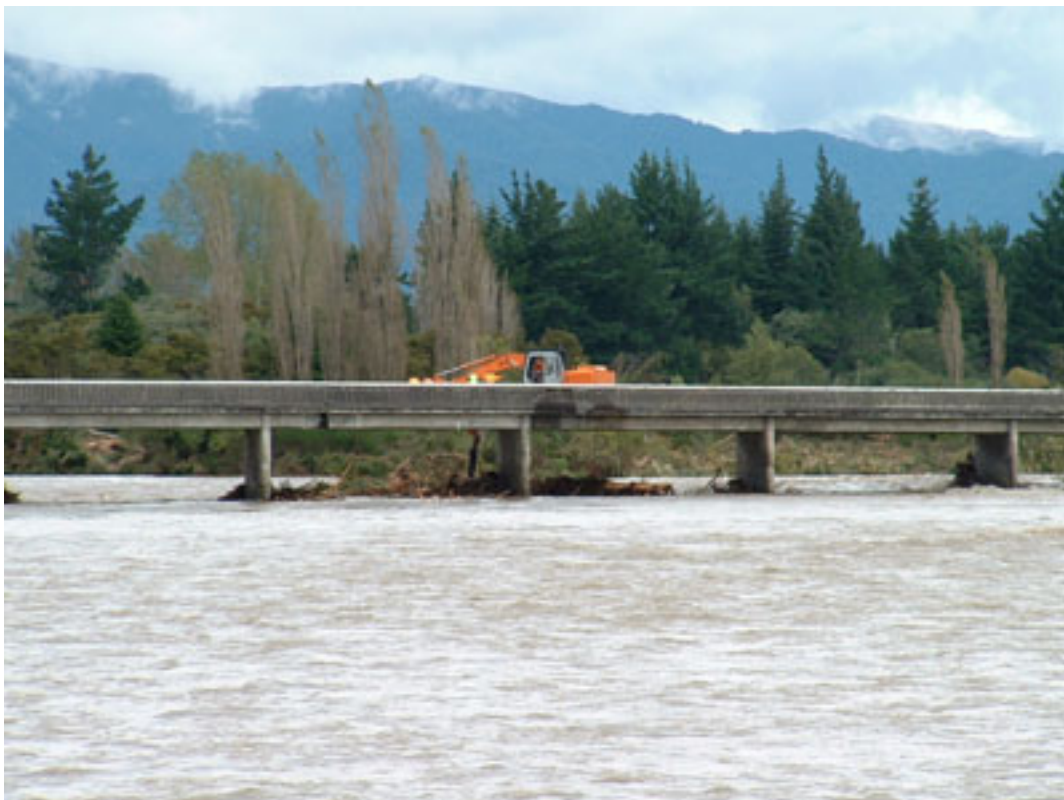
Figure 4 Typical multiple span road bridge during a high flow event
