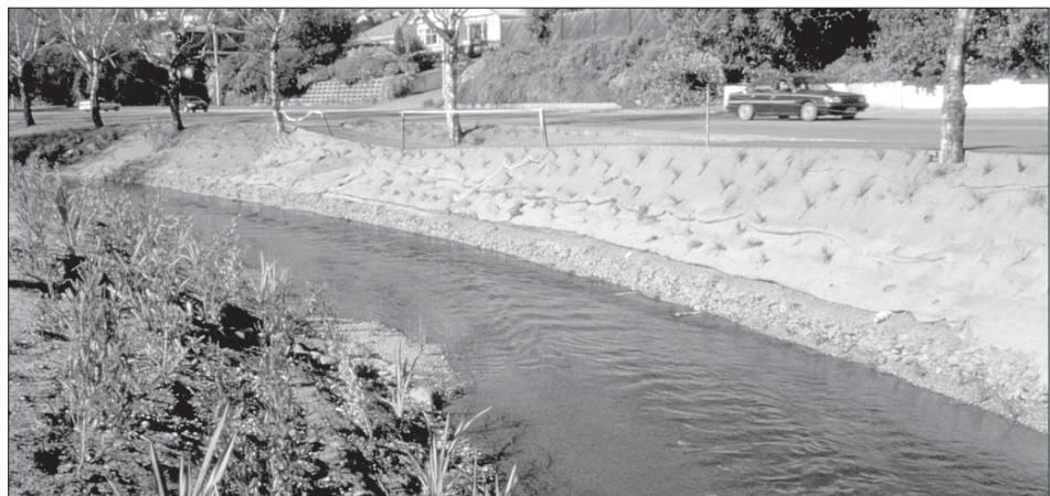
This wool mat on a steep river bank will suppress weeds, retain moisture and reduce erosion.
