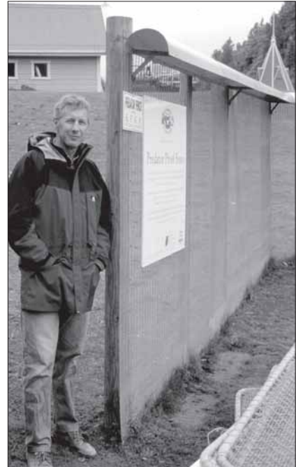
A demonstration section of the predator fence at the Karori sanctuary, Wellington. This elaborate fence even excludes mice and is also able to withstand human sabotage.
