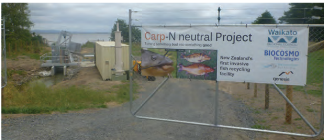
PLATE 4.4 Waikato Regional Council 'Carp-N neutral Project' demonstration site at Lake Waikare showing the carp separation cage structure in the fish pass channel with thermophilic digester to process captured invasive fish on the right.
