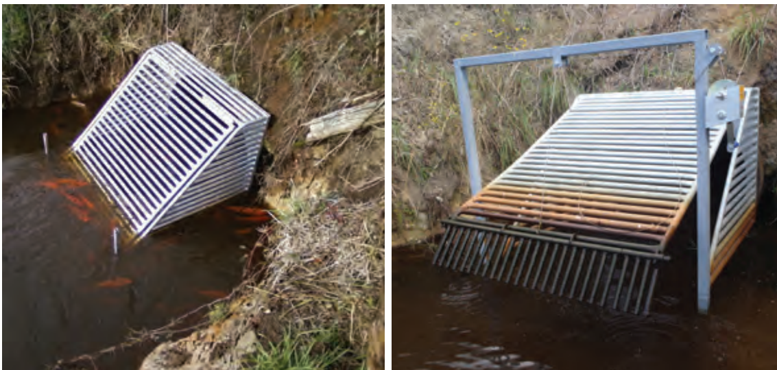
PLATE 4.7 Lake Ohinewai outlet drain fitted with a one-way gate showing adult koi carp attempting an upstream pass (left panel), and screen lifted for inspection and clearing of debris (right panel).
