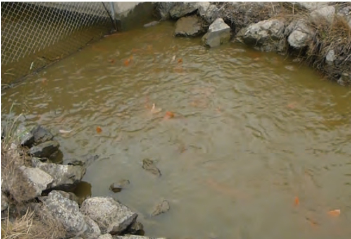
PLATE 4.6 Invasive fish accumulating in the Lake Waikare fish pass holding area having passed through the carp exclusion screen finger counter. Fingers are located underwater (below hurricane mesh). The Waikare carp separation cage is approximately 40 m upstream.
