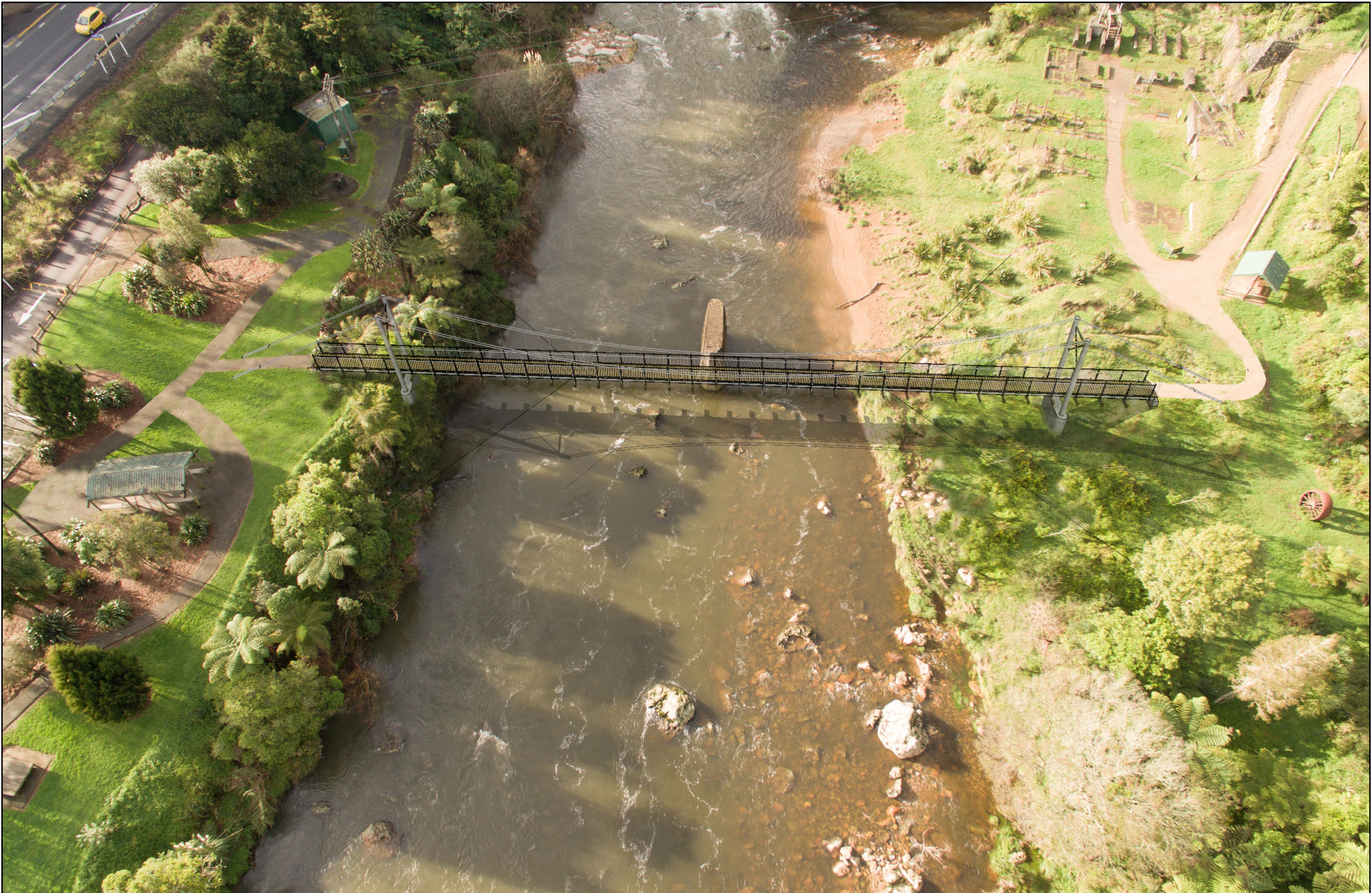
Ohinemuri Suspension Bridge Replacement 2018
