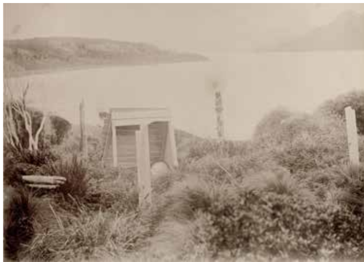
Figure 9. The remains of Epigwaitt hut in 1888, with the by-then derelict 1881 A-frame castaway depot that had been built by the crew of the Stella . Source: William Dougall Album, Canterbury Museum, 1982.86.3 .
