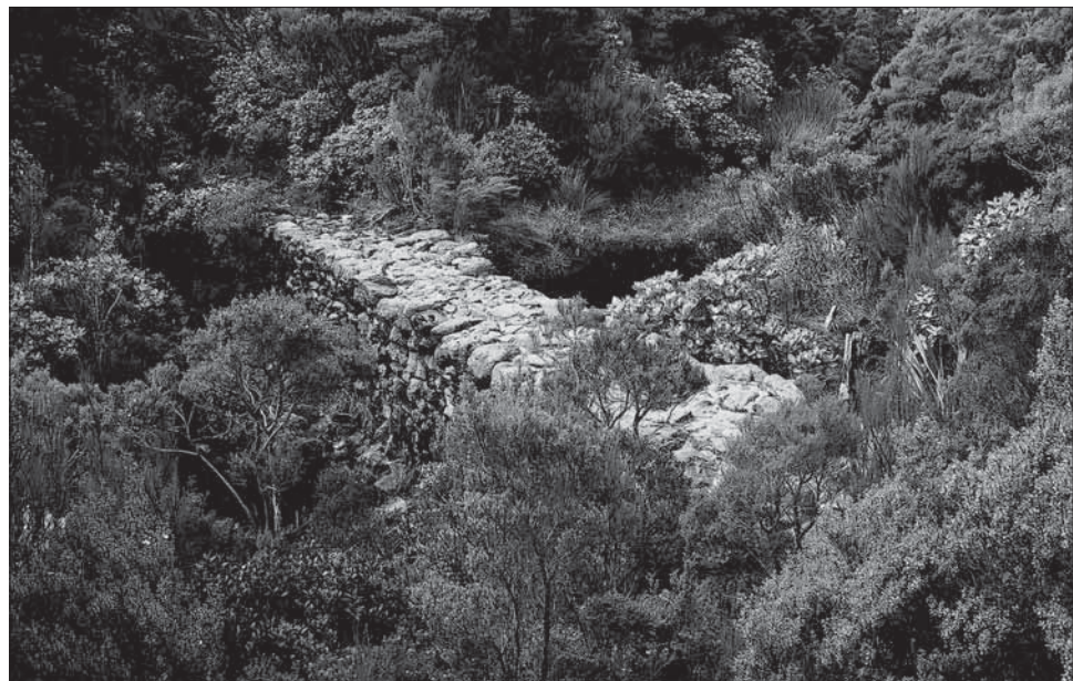
Figure 28. The stone dam (Site D49/38) in the headwaters of McArthurs Creek, built in about 1915 to supply the hydraulic sluicing operation. Photo: P. Petchey.
