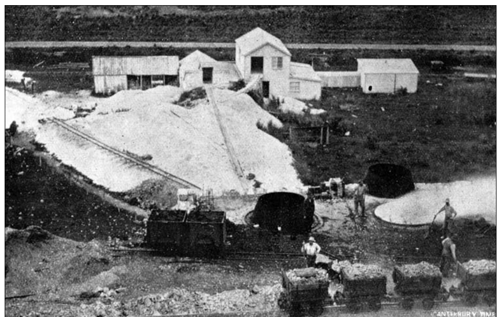
Figure 27. Lime kilns at Mount Somers, 1909. The tops of the bottle kilns are in the foreground. Lime was spread on fields to improve pasture quality. Photo courtesy of Canterbury Museum (Bishop Collection; reference number CMNZ 12795).
