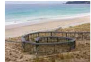
The pest-proof fence ends in a spiral. Traps in the centre of the spiral are set to catch animals running along the fence and prevent them entering the protected area. Photo: Lindsay Young
